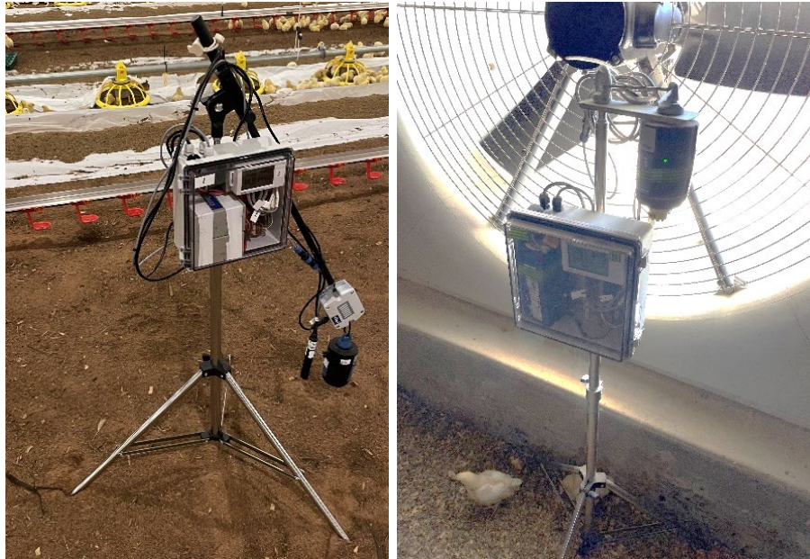
Figure 27. In-shed sensor stations (left – main in-shed sensor; right – the fan-stand).
