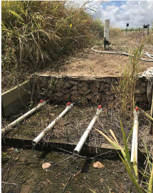
Figure 3.11 Outlet pipes.
