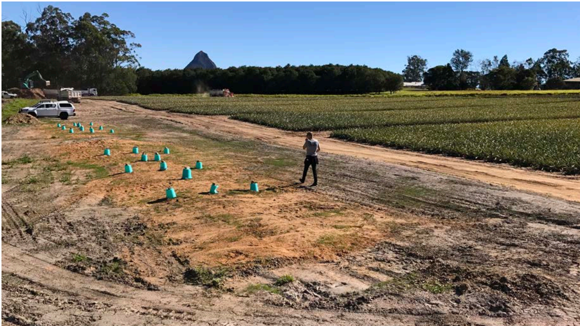
Figure 1.2 Bioreactor wall (i.e. under green buckets) installed downslope of a pineapple crop in South-East Queensland.
