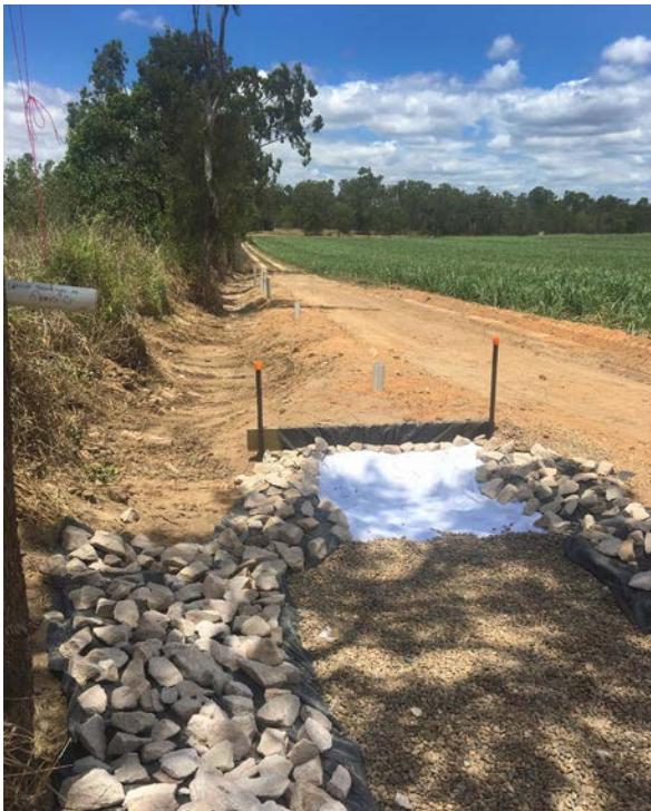
Figure 3.10 Gravel inlet pit (foreground).
