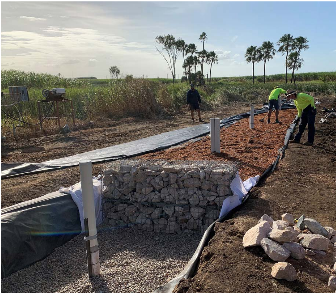
Figure 1.5 Spreading woodchip in a bioreactor bed.
