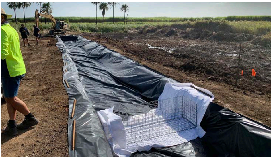
Figure 3.9 Bioreactor bed showing liner and gabion basket.
