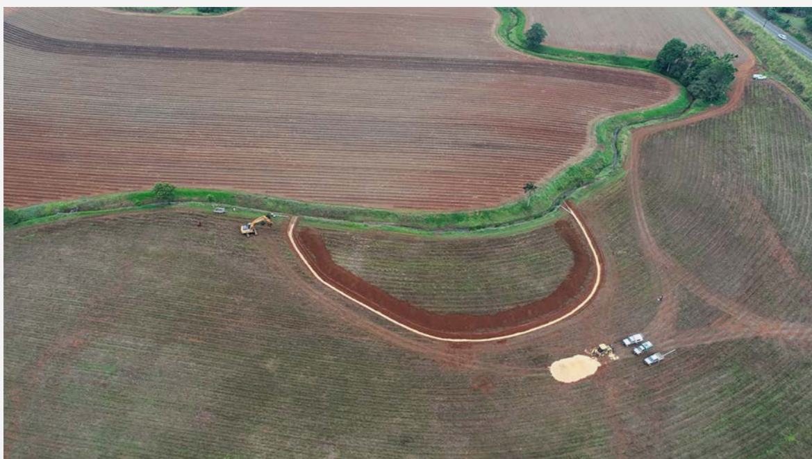
Figure 1 Aerial image of ag-pipe bioreactor under construction, showing cane crop and drainage line into which the bioreactor outlets. Source: WTMIP
