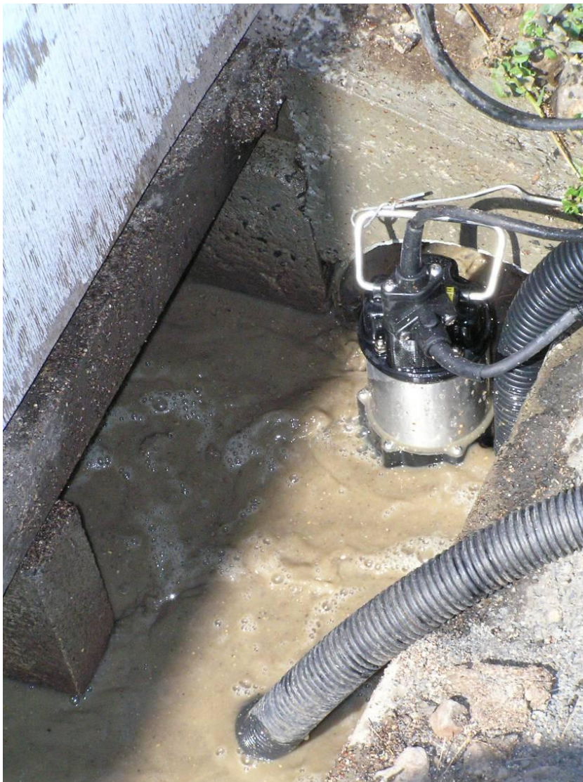
Figure 13: Pumped effluent sampling from the drain on the end of shed 4.
