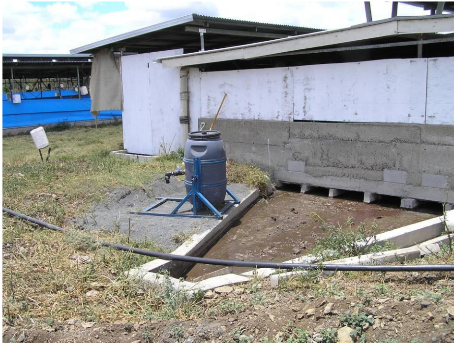
Figure 10: Tipping drum positioned for sampling from Shed 3.
