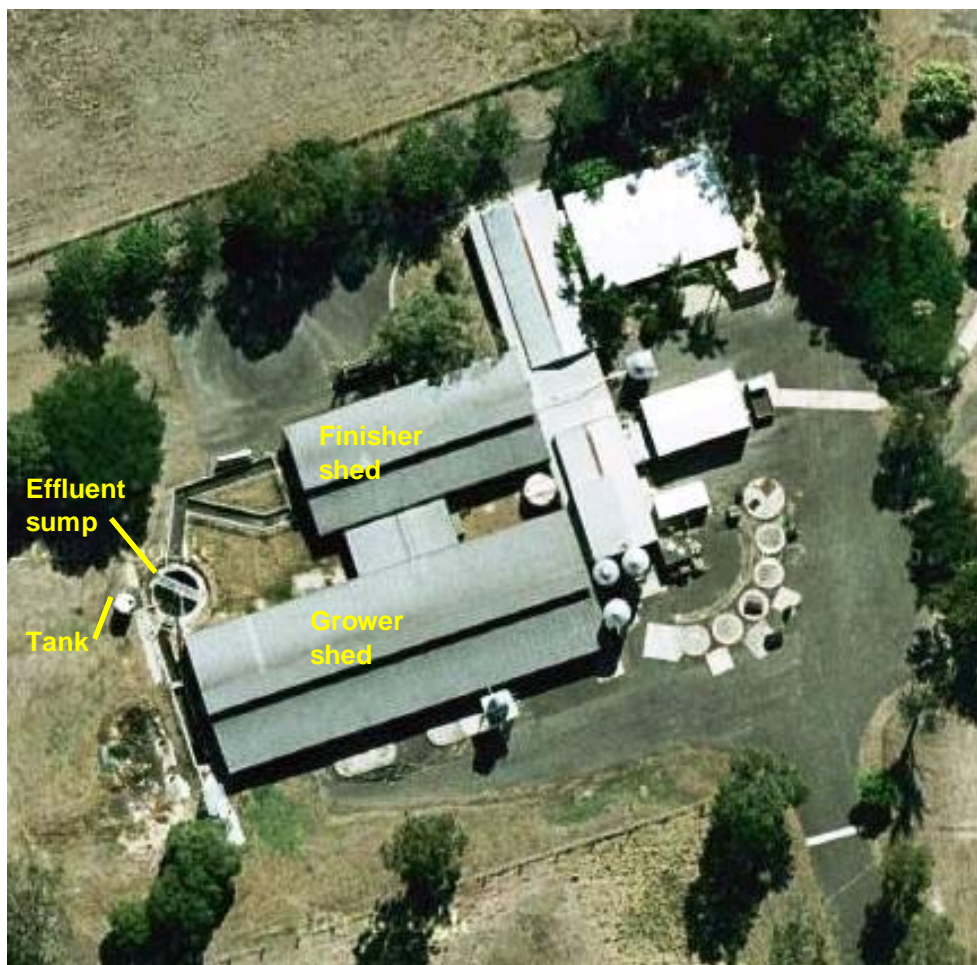
Figure 4: Grower and finisher sheds at the DPI&F Wacol piggery, showing the effluent sump and settling tank on the western end.
