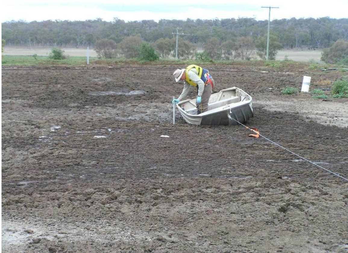
Figure 16: Using the aluminium tee-bar to estimate the depth to the top of the sludge layer that had accumulated on the base of the highly loaded pond at the Dalby piggery.
