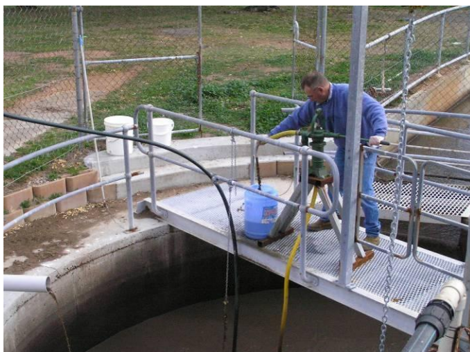
Figure 28: Collecting settling tank inlet sample using hand pump.
