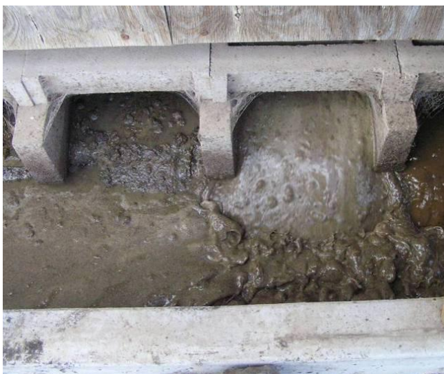
Figure 31: Initial discharge from one of the shed 5 flushing channels showing relatively high solids content.
