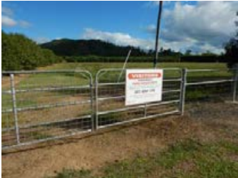
Perimeter fencing controls Movement of people and vehicles.
