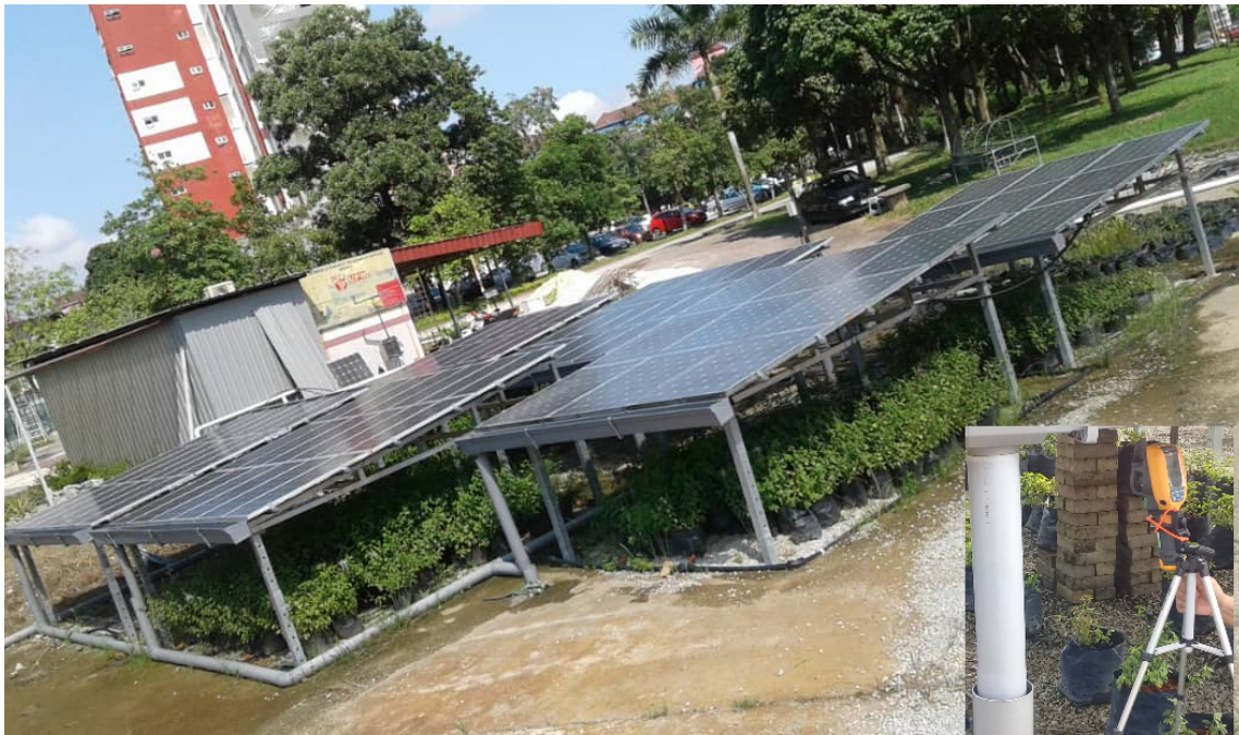
Figure 5. Agrivoltaic system with a Fluke thermal imager on a tripod for video recording.
