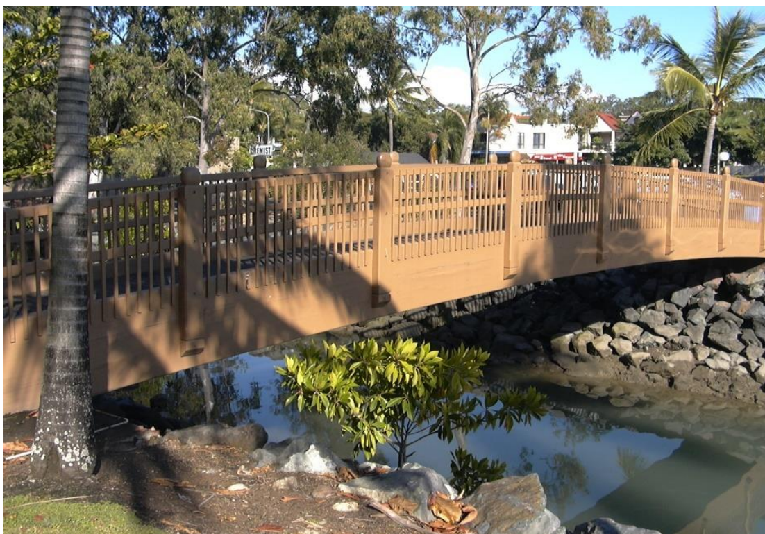
Figure 33. Glulam foot-bridge with protective finish. (Provided by Colin MacKenzie)
