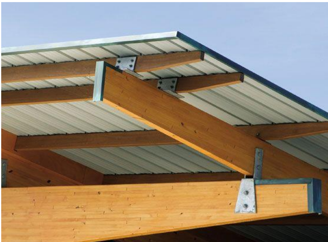
Figure 31. Capping protection of glulam in roof structure (Source – i.pinimg)
