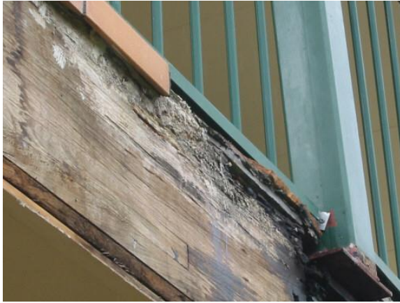
Figure 19. Decay in EWPs L and R. (Provided by Colin MacKenzie)
