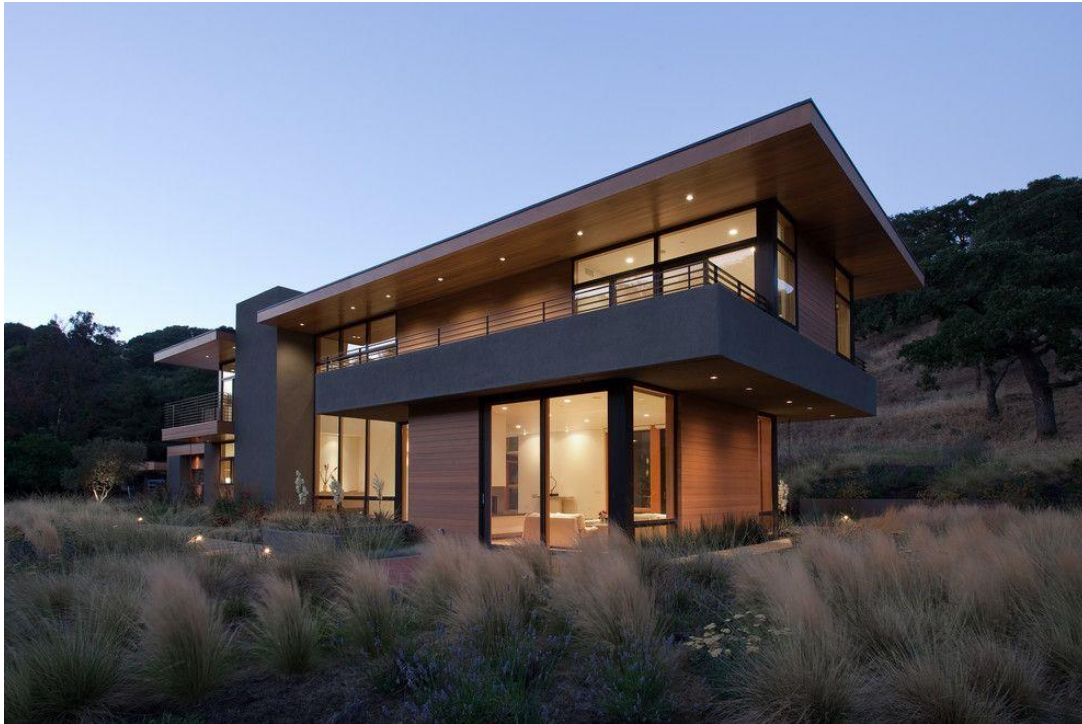
Figure 30. Large overhangs provide good protection against moisture ingress into buildings (Source – Better Home Lifestyle)
