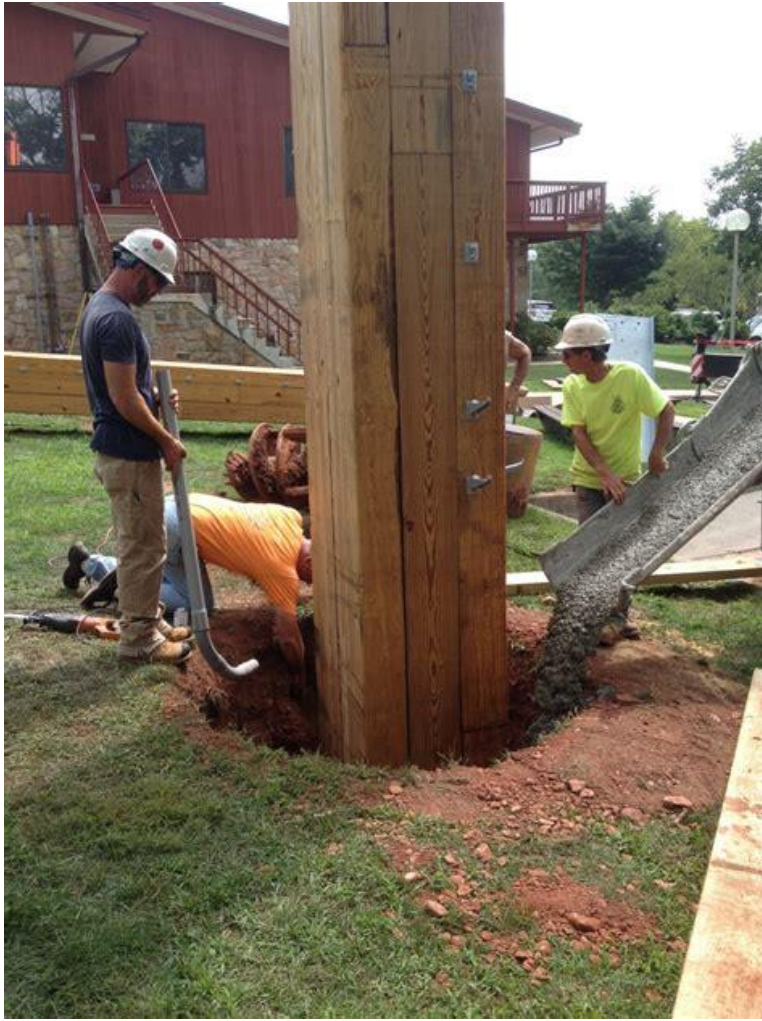
Figure 43. Installation of glue laminated utility pole (Source – New Jersey Business Systems, Inc.)
