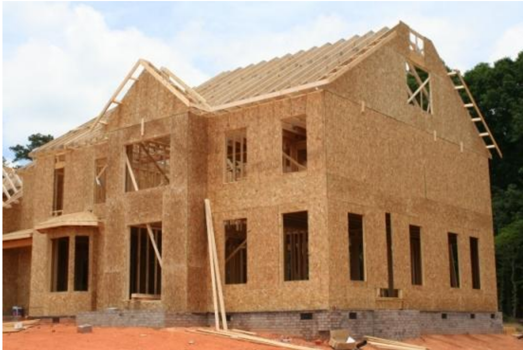
Figure 14. OSB used in house construction. (Source – IHB, 2018)
