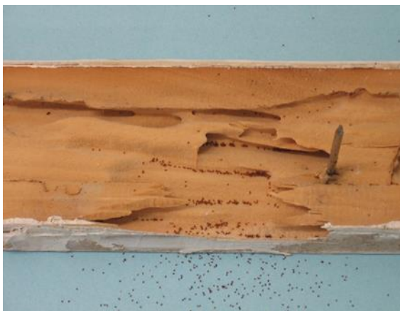
Figure 21. Termite damage to wood. (Source – DAF, Forest Products Innovation, 2017)
