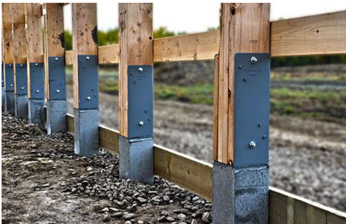
Figure 32. Glulam posts isolated from ground. (Source – Trout Creek Truss)
