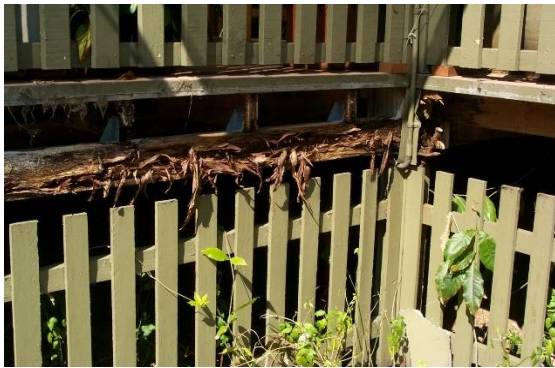
Figure 20. Further examples of decay in EWPs L and R. (Provided by Colin MacKenzie)
