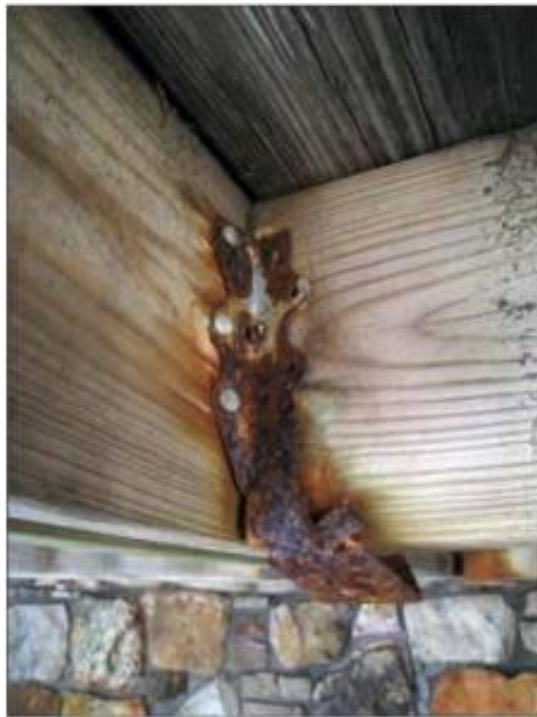
Figure 24. Corrosion of metal fasteners in wood. (Source – Carpentry Contractor Blog (L) and Forest Products Lab, USDA Forest Service, 2015)
