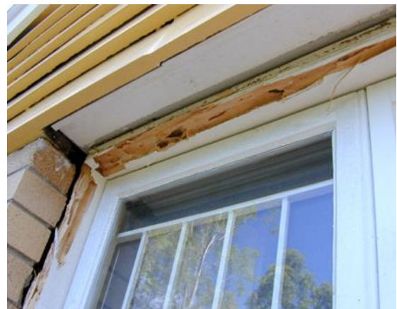
Figure 21. Termite damage to wood. (Source – DAF, Forest Products Innovation, 2017)
