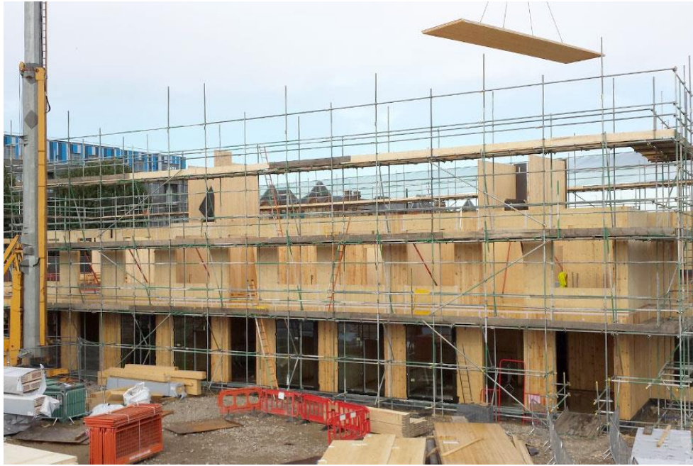
Figure 6. CLT being used in building construction. (Source – Avanti Architects, 2017)
