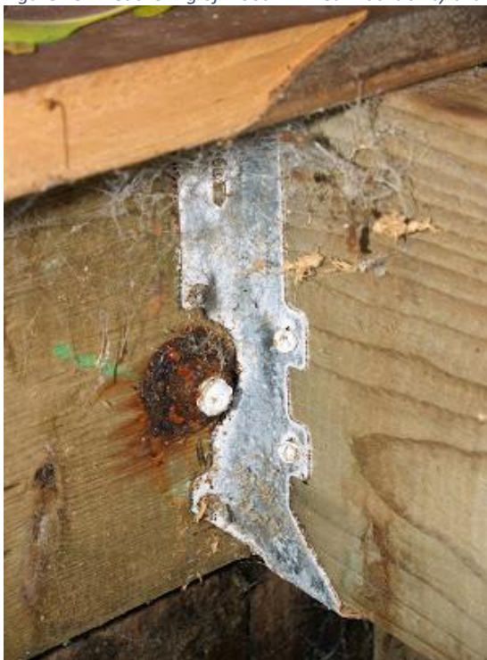
Figure 24. Corrosion of metal fasteners in wood. (Source – Carpentry Contractor Blog (L) and Forest Products Lab, USDA Forest Service, 2015)
