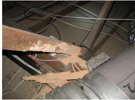
Figure 22. Lyctid beetle (borer) damage to wood including larvae and frass. (Source – Doug Howick (L) and Ted Stubbersfield (R)).
