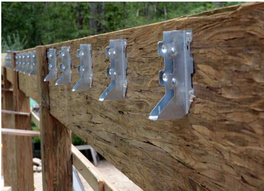
Figure 16. Pressure treated Parallam Plus. (Source – Weyerhaeuser, 2018).
