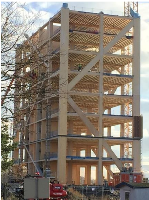
Figure 4. Glulam structure in construction in Norway
