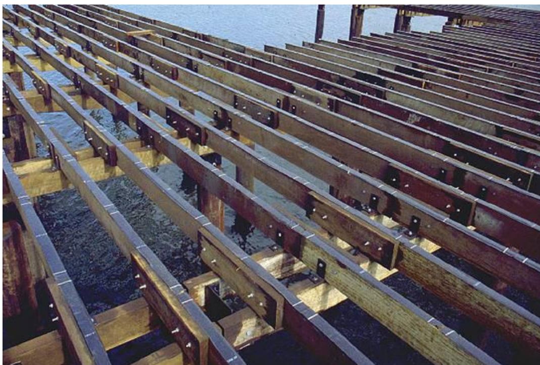
Figure 34. Bituminous Damp Proof Course (DPC) fixed to top of deck joists. (Provided by Colin MacKenzie et al., 2015)
