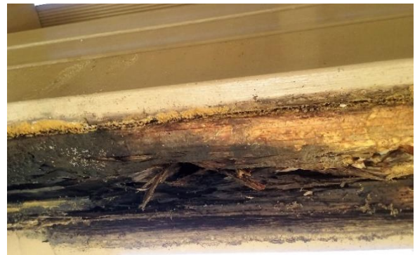
Figure 20. Further examples of decay in EWPs L and R. (Provided by Colin MacKenzie)
