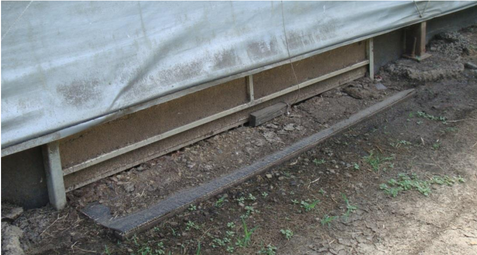
Figure 11. 'Pop-hole' on the wall of a free-range shed that is opened to allow the birds access to the range
