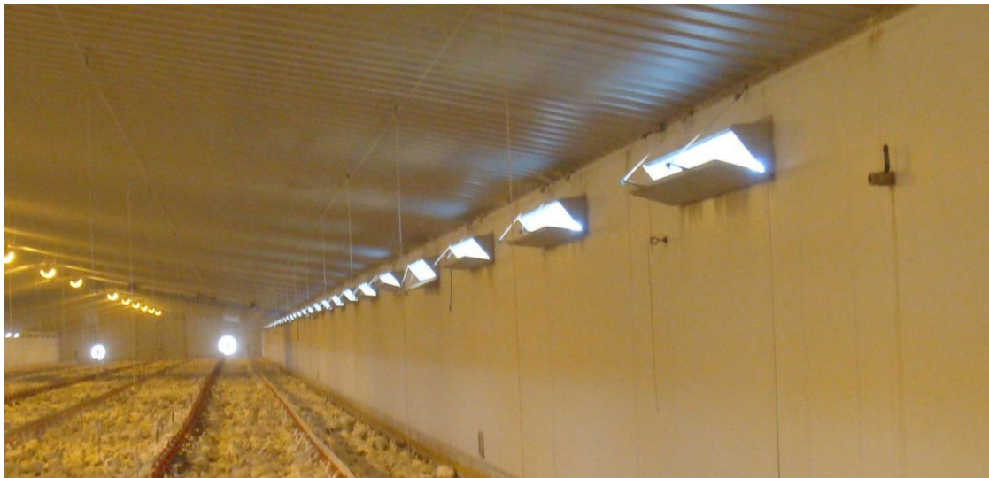
Figure 7. Mini-vents as viewed from the inside of the shed. These mini-vents are open to allow air to enter the shed.
