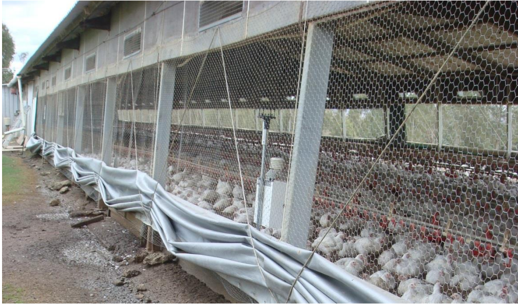
Figure 10. Naturally ventilated sheds have curtains or flaps on the walls that are opened or closed to maintain the correct conditions within the shed.
