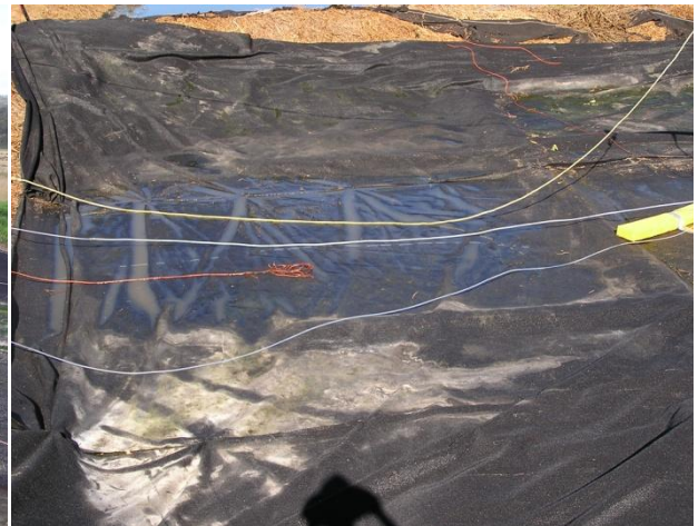
vi) Cover after 16 months (June 2004); shade cloth installed
