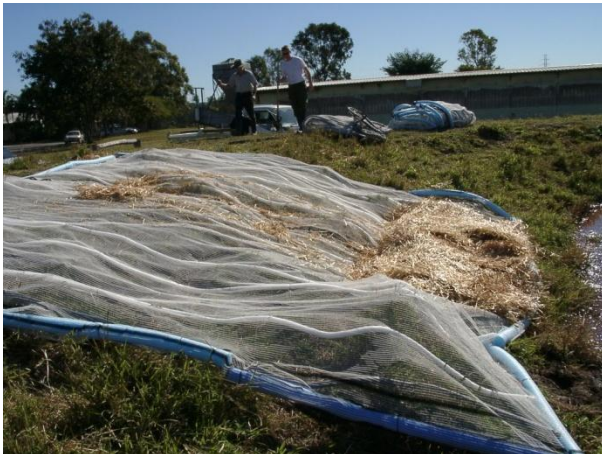
Figure 85: Trial supported straw cover, manual application of straw on pond margin
