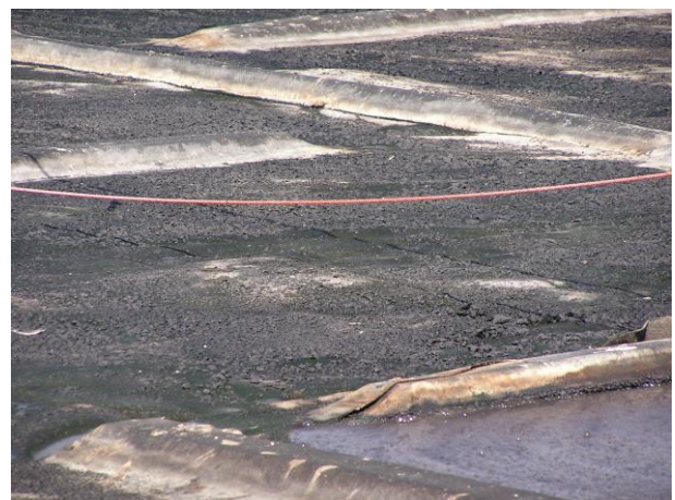
Figure 124: Biomass drying on cover surface to form dried cake
