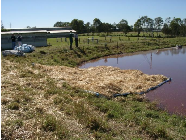
Figure 87: Trial supported straw cover, manual application of straw 3
