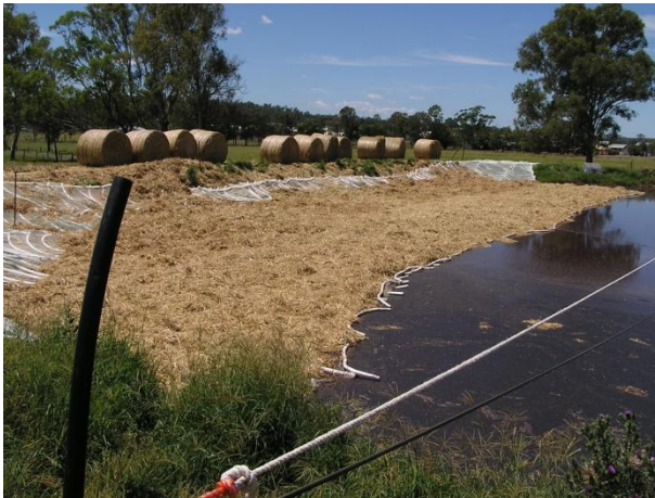
Figure 91: Full-size supported straw cover, manual application of straw 3
