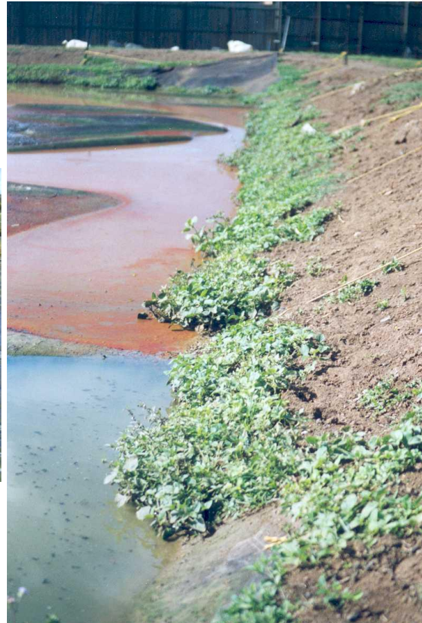
Figure 109: Permeable pond cover some time after installation – note submersion of cover along margin following erosion of bank material.
