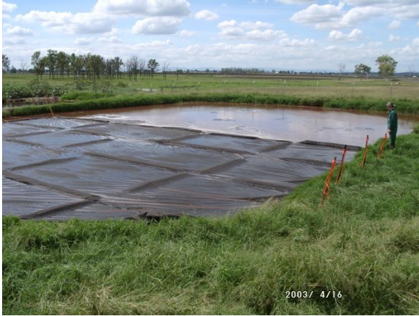
Figure I01: Deployment of polypropylene cover 2
