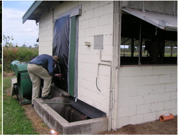
Figure 18: Making a leak-tight connection between shed doorway and fan
