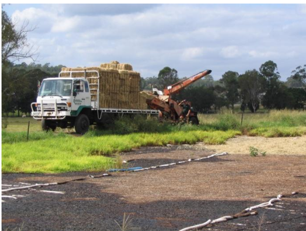
Figure 95: Mechanical application of straw to supported cover 1
