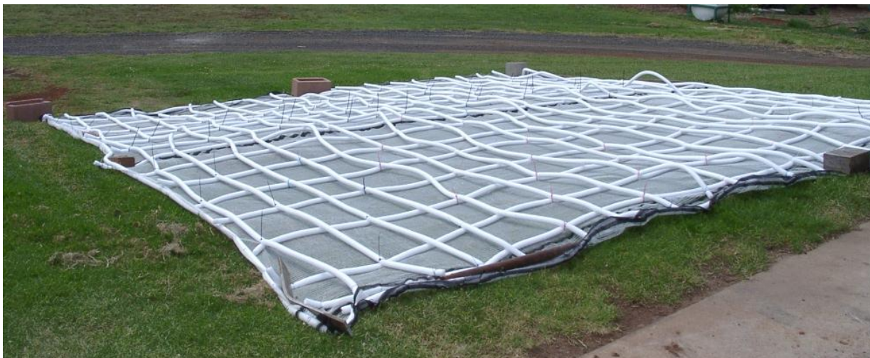
Figure 83: Straw support materials – hail netting and backer rod.
