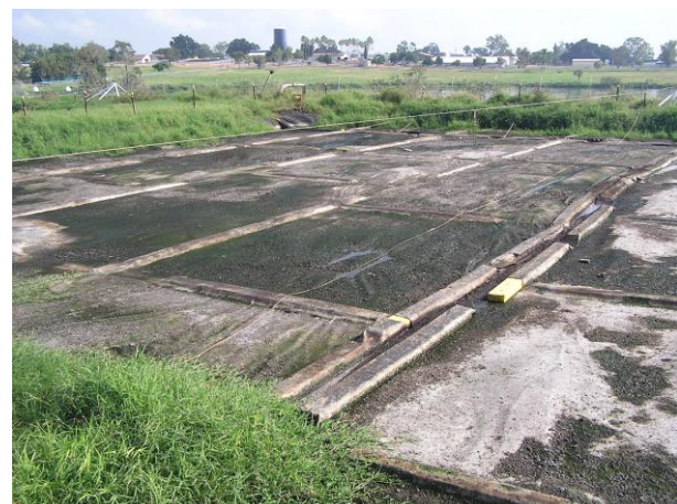
Figure 116: Encroachment of couch grass onto cover 12 months after deployment
