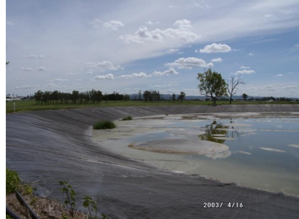
Figure 118: Water ponded on surface of impermeable cover
