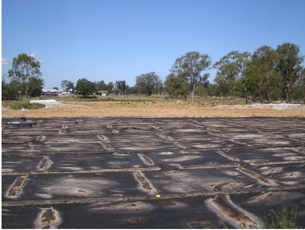
Figure 93: Full-size supported straw cover, manual application of straw 5
