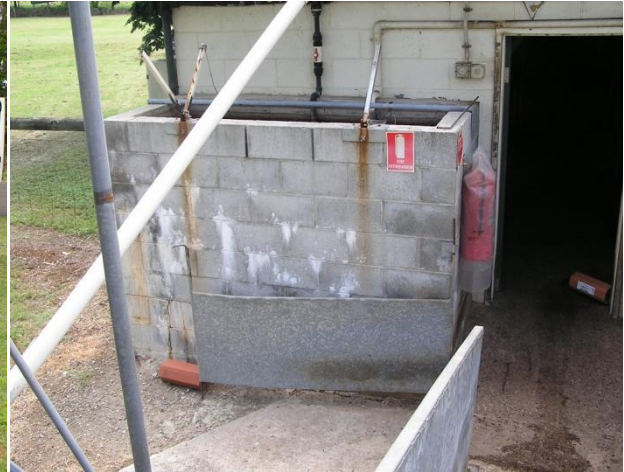
Figure 21: Concrete flushing tank on opposite end of shed to that used for odour sample collection
