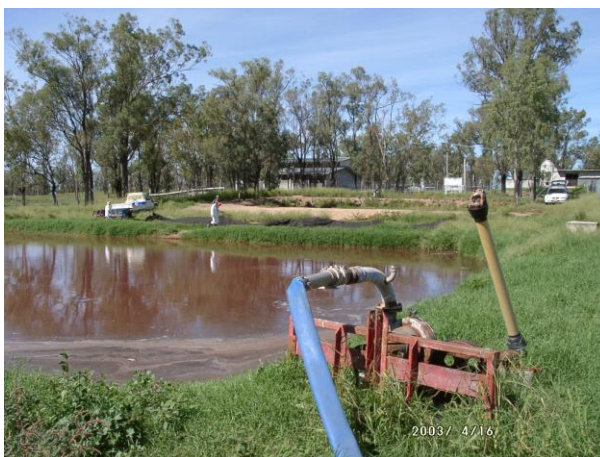
Figure 115: Encroachment of couch grass onto pond prior to deployment of polypropylene cover
