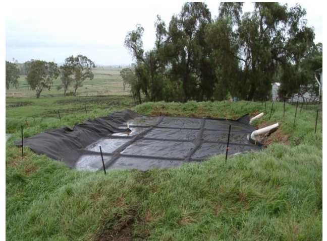
Figure 2: Polypropylene cover deployed on pond
