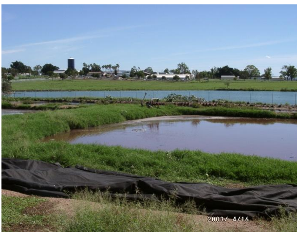
Figure 3: Polypropylene cover ready for deployment
