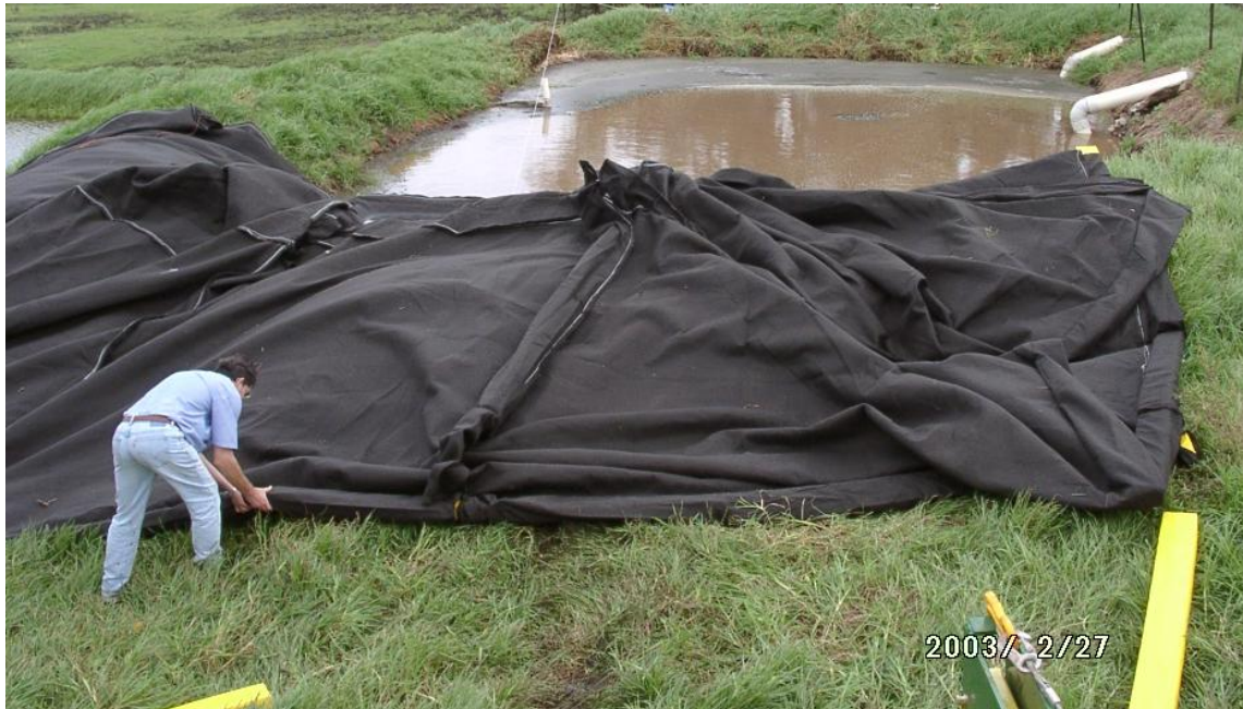
Figure 84: Inserting Canvacon® covered polystyrene rods into pockets in the polypropylene cover.
