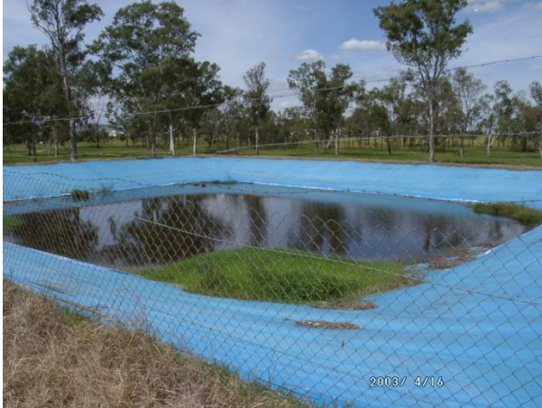
Figure 117: Water ponded on surface of impermeable cover
