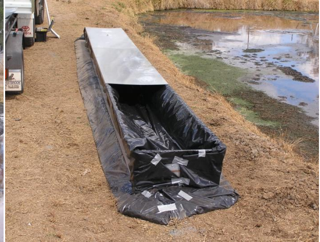
Figure 14: Partially constructed lined flume looking down-gradient
