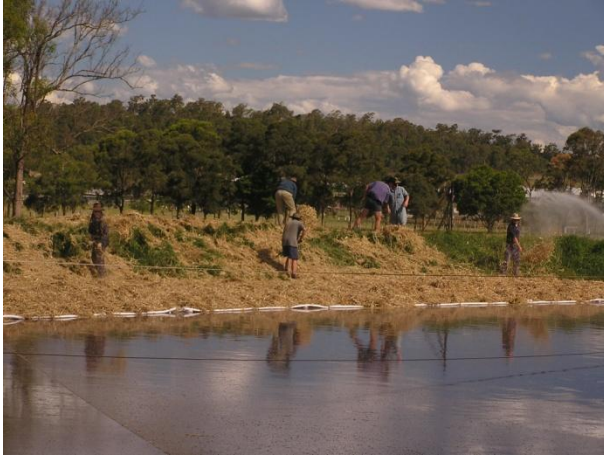
Figure 90: Full-size supported straw cover, manual application of straw 2
