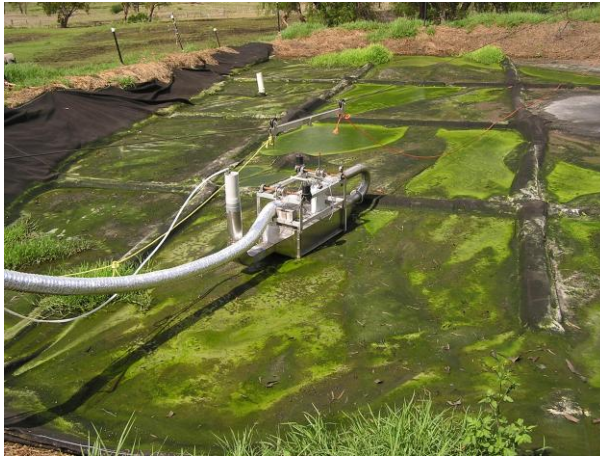
Figure 119: Water ponded on surface of permeable cover 1
