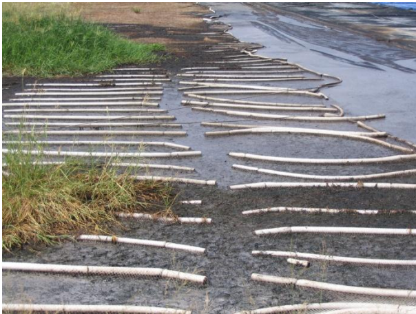
Figure 94: Degradation of straw 15 months after manual application of straw
