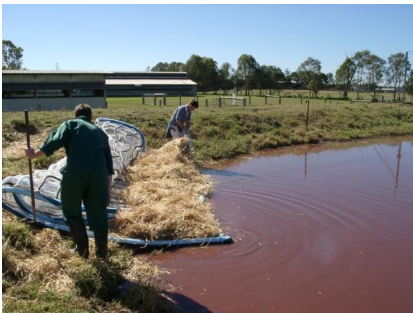
Figure 86: Trial supported straw cover, manual application of straw on pond margin
