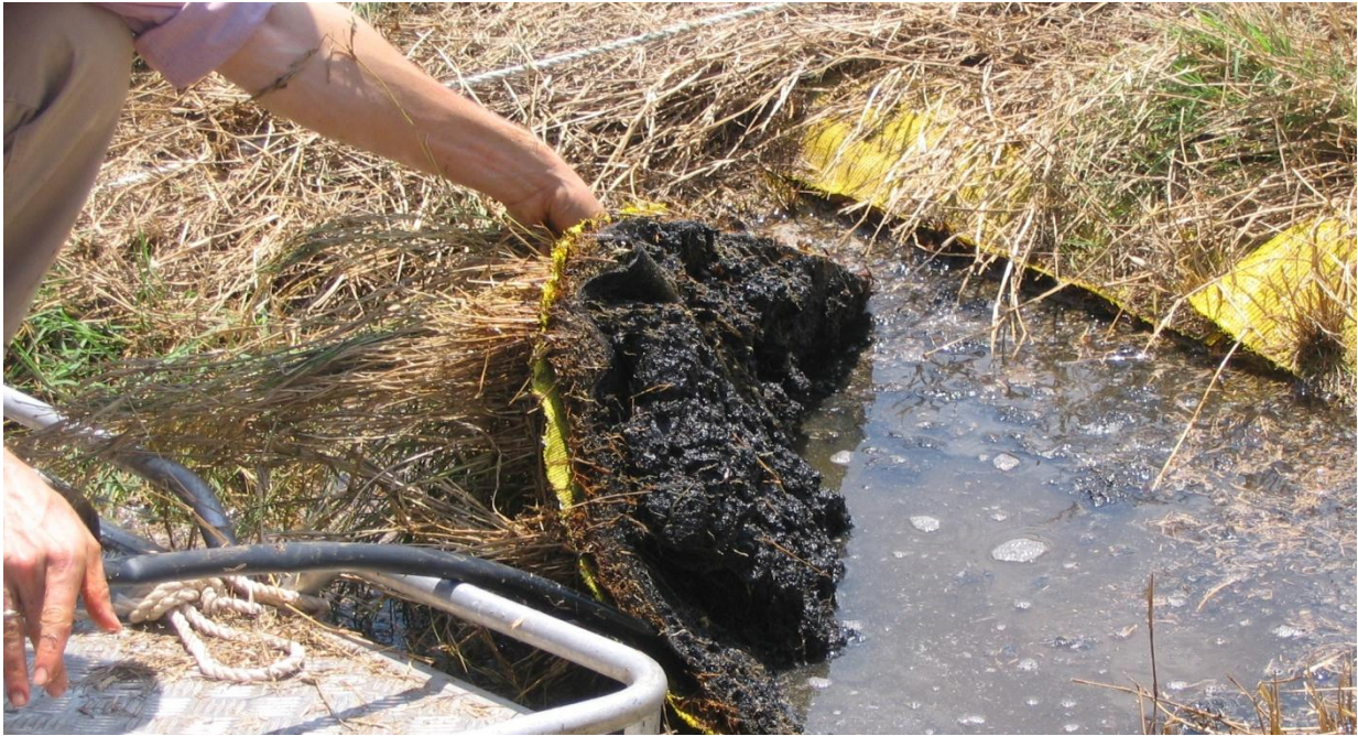
Figure 38: Extensive growth of roots of couch grass through the pond cover (piggery C)
