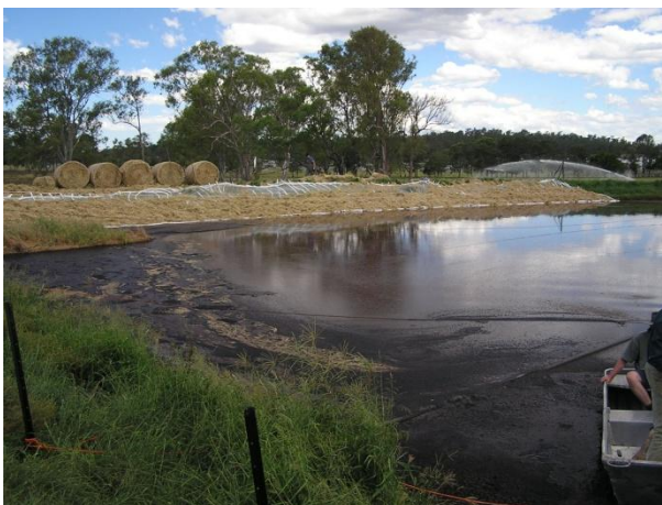
Figure 89: Full-size supported straw cover, manual application of straw 1
