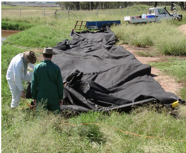
Figure 100: Deployment of polypropylene cover I
