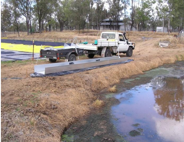
Figure 13: Partially constructed, unlined flume looking down-gradient
