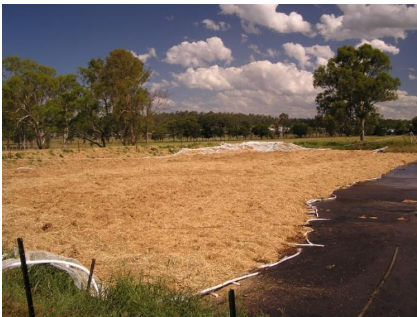
Figure 92: Full-size supported straw cover, manual application of straw 4
