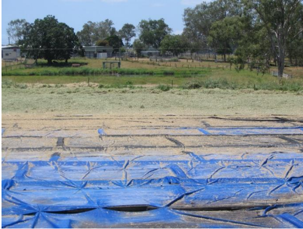
Figure 99: Refurbished supported straw cover
