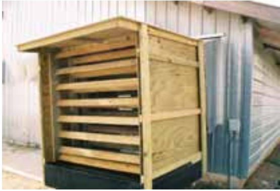
Figure 19 USDA-ARS ammonia scrubber installed on a broiler shed ventilation fan, from (Moore et al., 2006)
