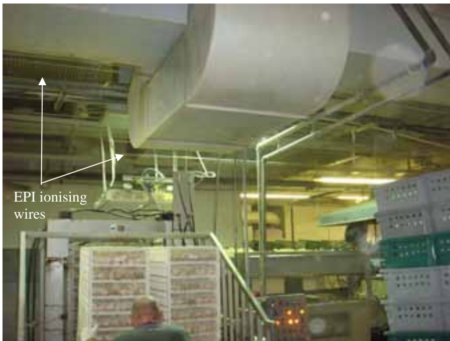
Figure 30 Turkey hatching room where the EPI system was installed (EPI ionising wires are visible above the machinery)
