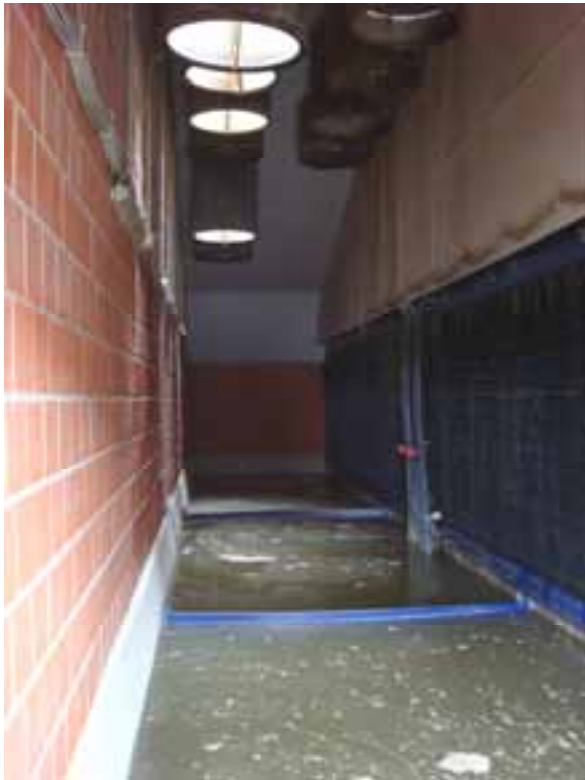
Figure 13 MagixX system installed in a poultry house in Germany - rear view of filter bank showing proximity to the rear wall and roof mounted ventilation fans
