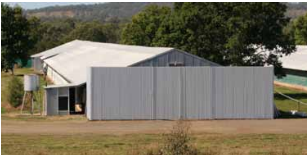
Figure 37 Windbreak wall constructed at a broiler farm
