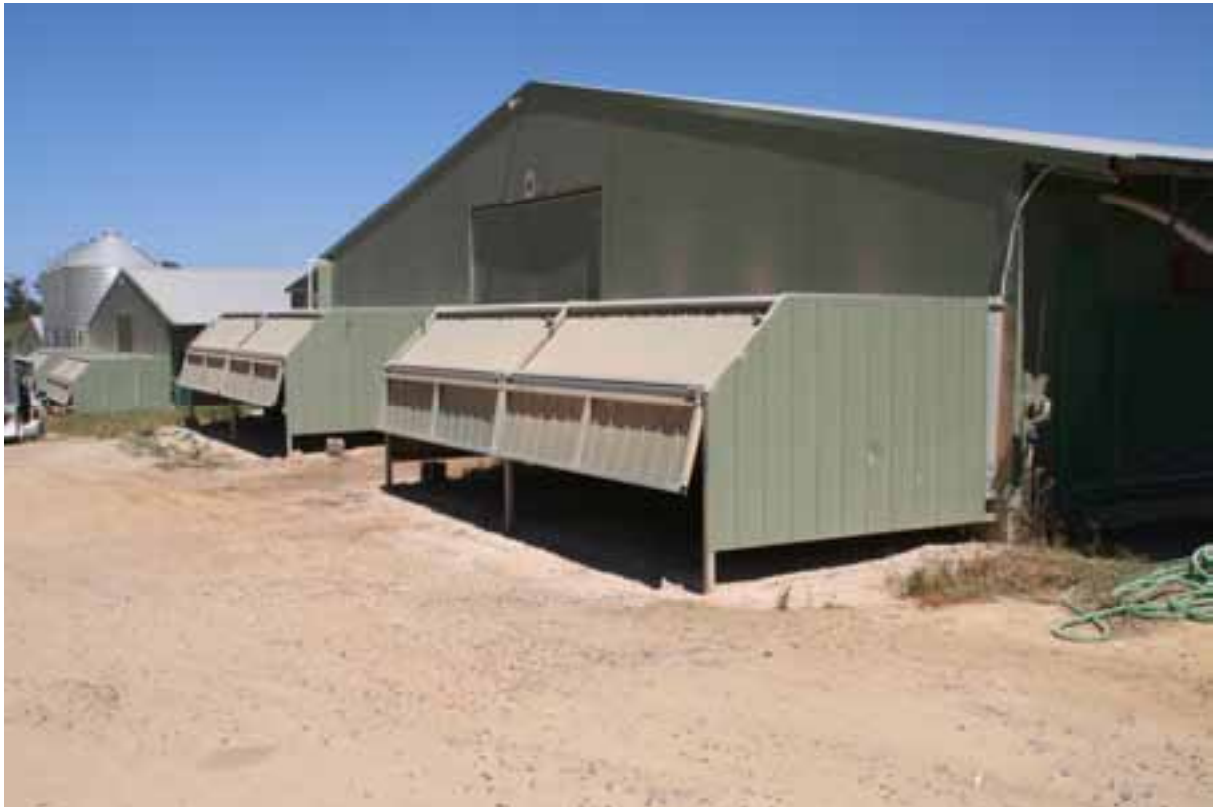
Figure 34 Grouped fan hoods placed over tunnel ventilation fans to direct dust and feathers downward
