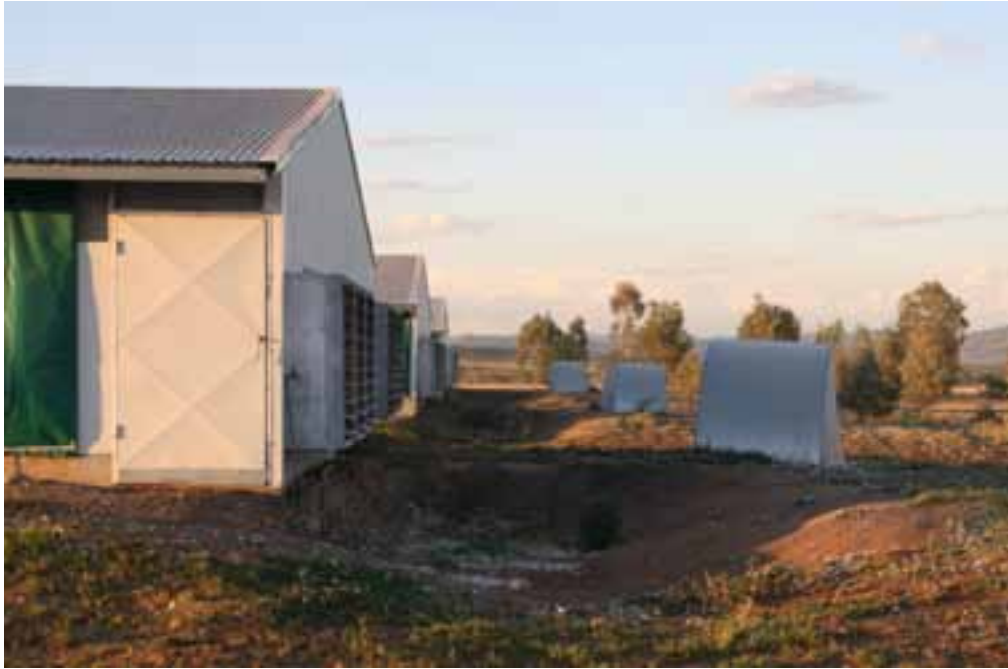
Figure 40 Excavation under fans to improve fan performance when hoods were fitted
