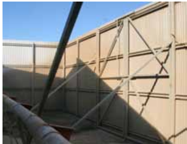
Figure 39 Dust on the windbreak wall 15 days after construction (birds aged 28 to 43 days during this period)
