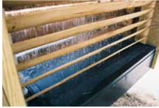
Figure 19 USDA-ARS ammonia scrubber installed on a broiler shed ventilation fan, from (Moore et al., 2006)
