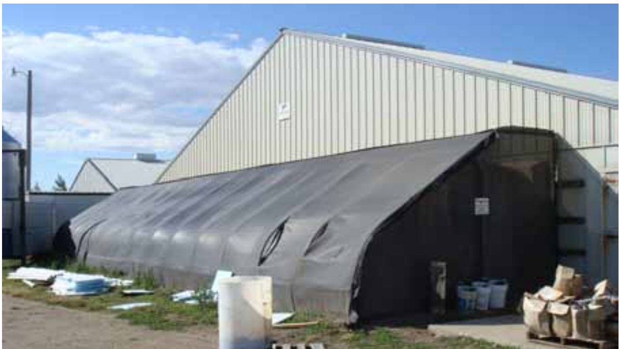
Figure 41 BioCurtain® installed on a pig shed in Minnesota, USA
