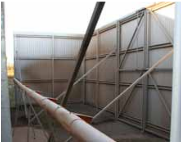
Figure 38 Dust on the windbreak wall 5 days after construction (birds aged 28 to 33 days during this period)
