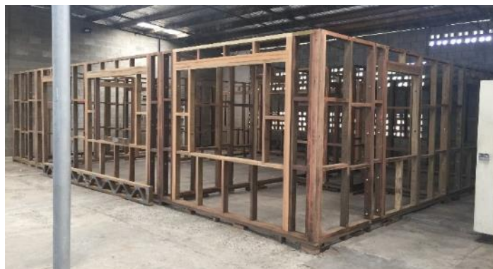
Figure 17: Pre-fabricated modular housing prototype at Omni Limited in Port Moresby.
