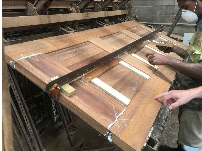
Figure 10: Door fabrication at LBC using new single component polyurethane adhesive.
