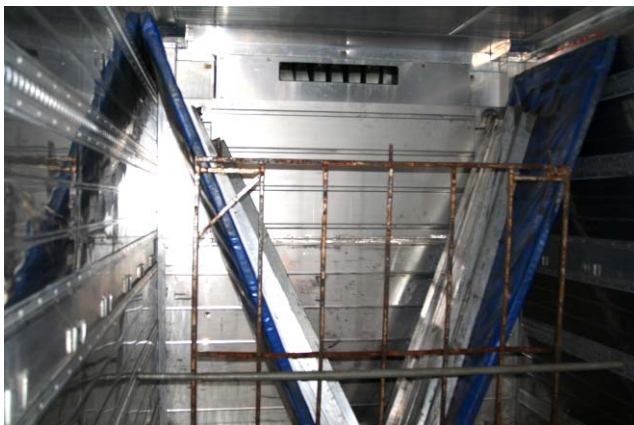
Plate 31 The gap between the front of the container and the first row of pallets. The spreader bar and grate maintains the 1m gap between the front of the container and the first row of pallets.
