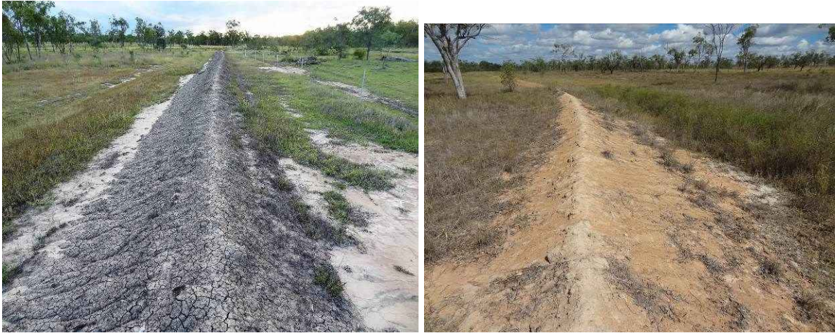
Image 15. L. Diversion bank to keep creek overflow off experiment site at Spyglass; and R. Contour bank protecting site from hillside water wash.
