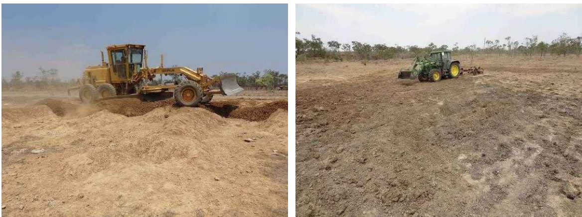
Image 12. L. Grader battering break-away gully head; and R. Crocodile plough seeder sowing grasses and legumes for hay mulch treatment at Spyglass (Oct. 2011).
