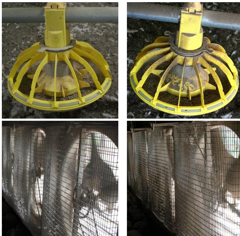
Figure 12. Dust accumulation on day 45 of a grow-out in control sheds (left) and sprinkler sheds (right) on feed pans and fan grills. Sprinkler position were later changed near the fans to reduce dust accumulation
