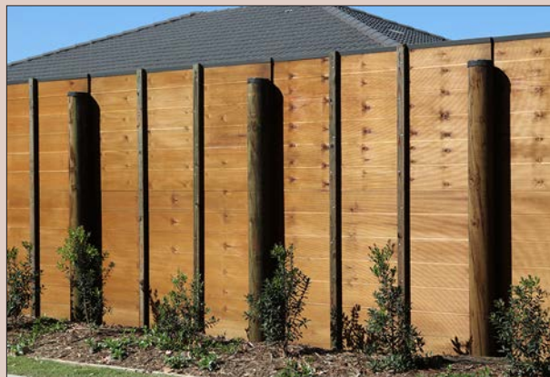
Figure 11.5. Preservative-treated plywood used for noise barrier construction.
