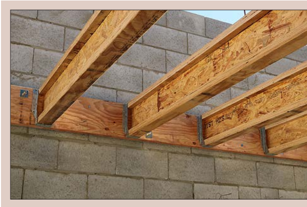
Figure 2.6. Structural beams combining rotary veneer flanges and oriented strand board web.
