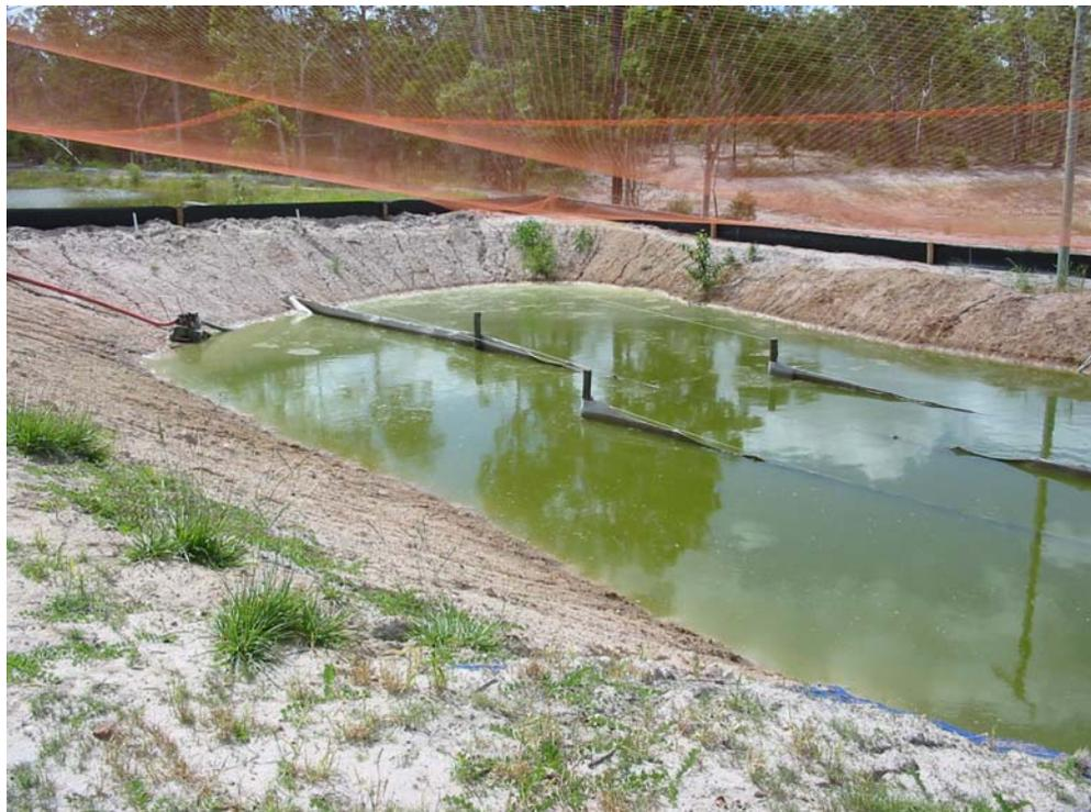
**Figure 8.3.** The 300m<sup>2</sup> treatment pond was partitioned to encourage directional water flow to maximize solids settlement and treatment of wastes.
