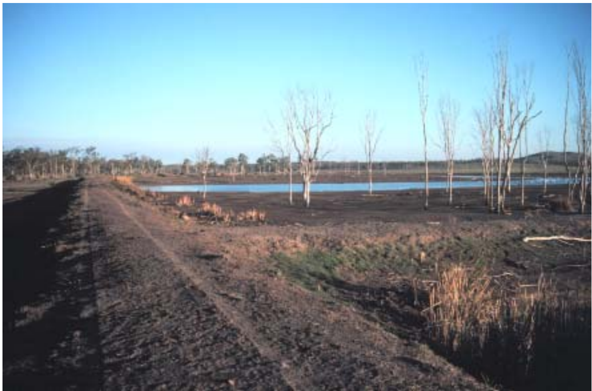
Pondage System in Fitzroy Estuary
