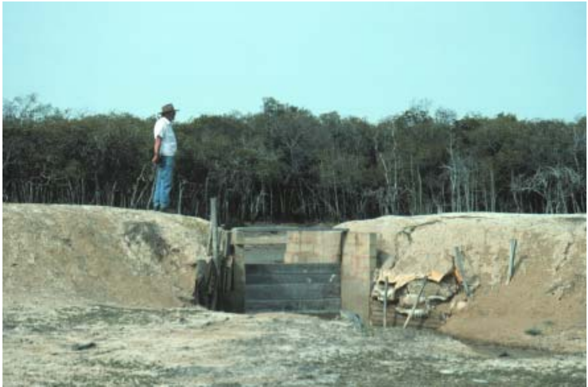
Pondage bank with sluice gate adjacent to mangroves, Broad Sound.
