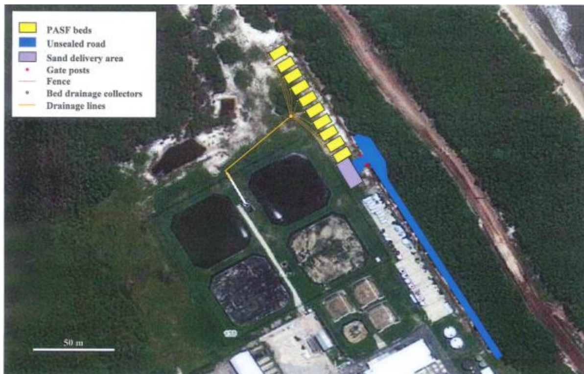
Figure 1 Aerial view of BIRC showing position of PASF development.
