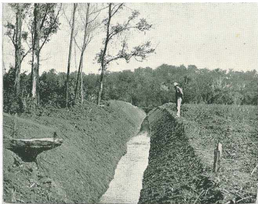
MAIN DRAIN, PETRIE'S CREEK.
