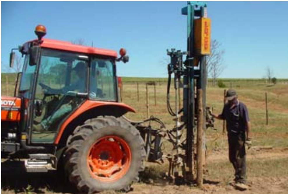
Figure 16: Installation of posts at Seppelt Winery, Great Western
