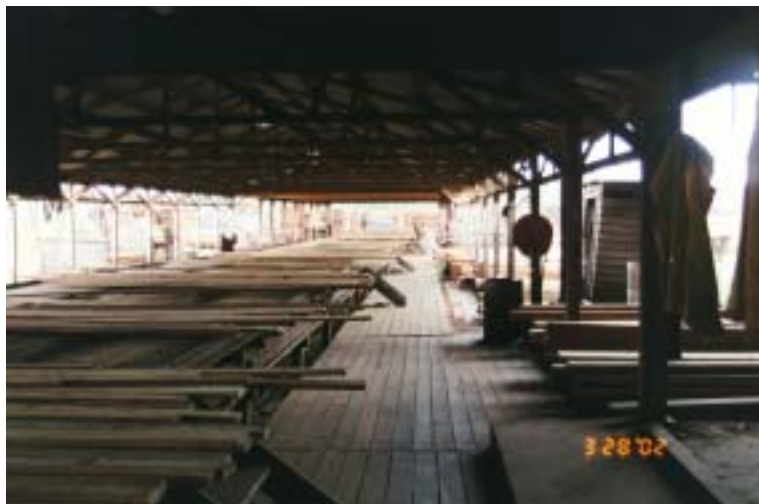
Figure 4.06. A covered linear green grading chain. The racking and stacking positions are exposed to the weather
