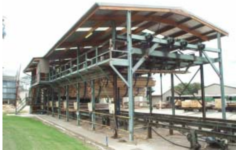
Figure 4.09. A pocket sling sorter. Boards of the same grade and dimension are assembled into groups before progressing to a stacker or racking machine
