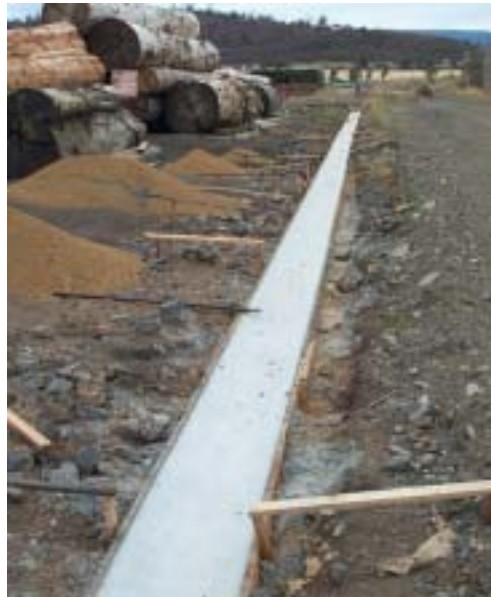
Figure 3.08. Spoon drain being installed in a log yard
