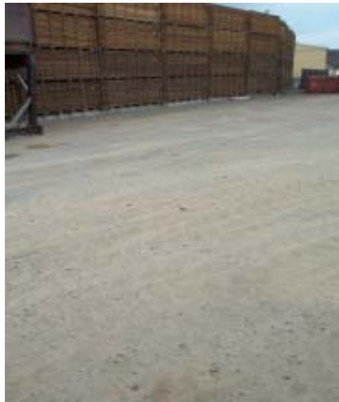
Figure 3.04. Firm and dry gravel hard standing
