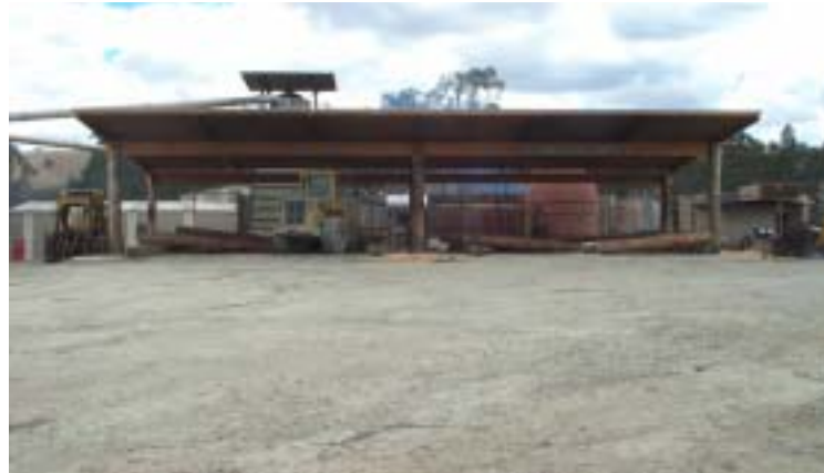
Figure 3.10. Shelter over log preparation area
