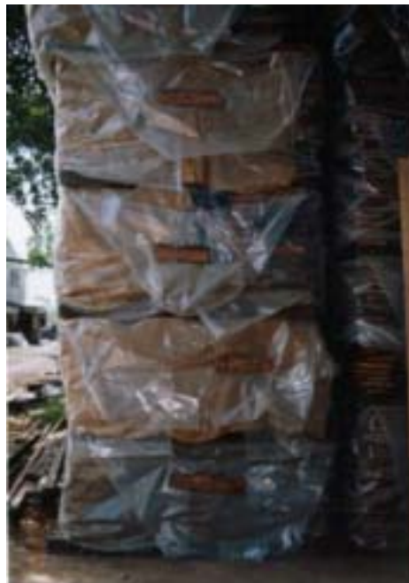
Figure 7.11. In adverse environments, drying can be slowed by local environmental control
