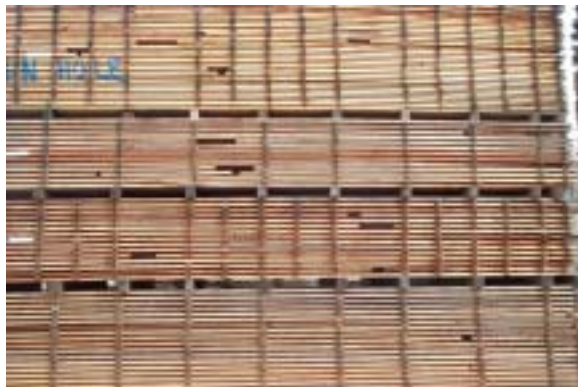
Figure 7.40. Desirable: Bearers and gluts in line
