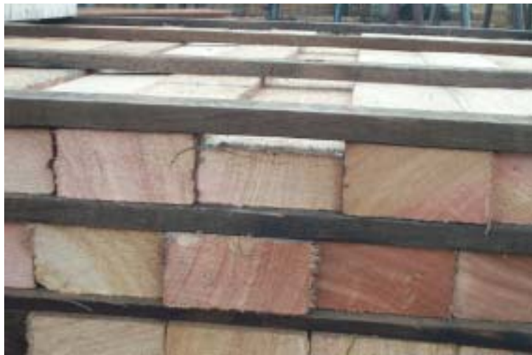
Figure 4.01. Result of poor cutting
