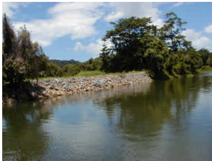
Plate 3. Rock wall constructed on the Russell River to minimize erosion.
