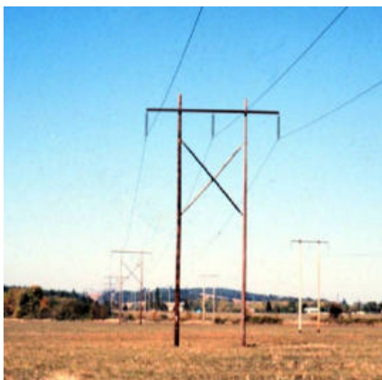
Figure 29 Typical softwood H-frame in-service in the USA (Courtesy Prof. Jeff Morrell, Oregon State University)
