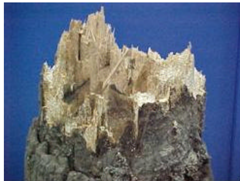
Figure 39 Example of white rot in a timber pole
