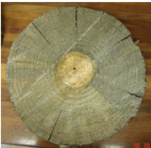
Figure 4 Typical distribution of untreated heartwood (yellow) and treated sapwood (grey-green) in a P. elliotii pole
