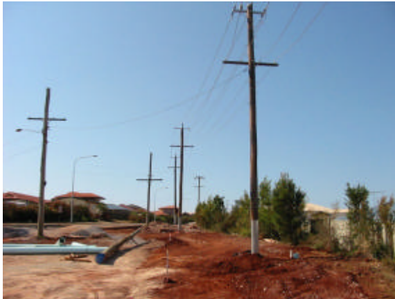
Figure 27 Newly installed rebuttet poles (courtesy Mr Doug Cowey, Pole Rebutters Australia)
