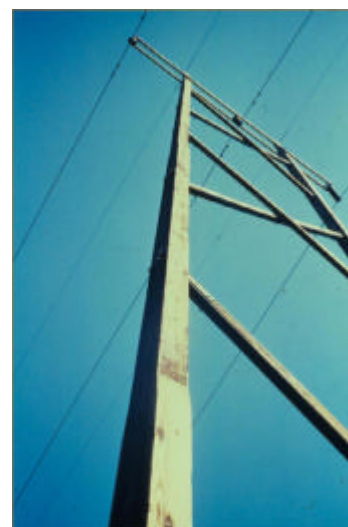
Figure 29 Typical softwood H-frame in-service in the USA (Courtesy Prof. Jeff Morrell, Oregon State University)
