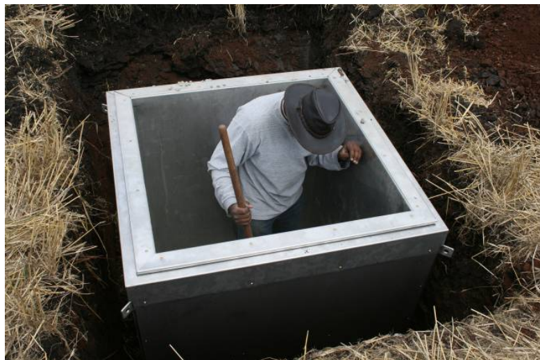
Figure 47. Installing lysimeters at Kingsthorpe (13 Nov 2008).
