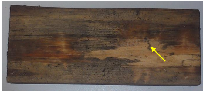
Figure 6 Discolouration caused by incipient (early) decay on the underside of a pine control specimen exposed at the South Johnstone field test site
