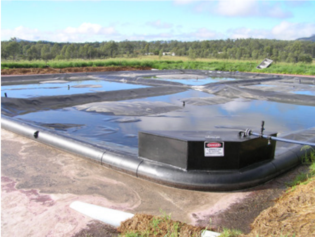
Figure 26. Floating pond cover installed on piggy anaerobic effluent pond.
