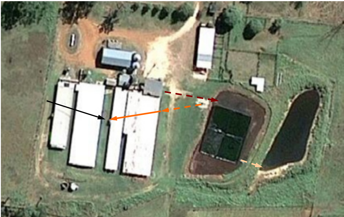
Figure 25. Aerial view showing piggery sheds and partially covered pond.
