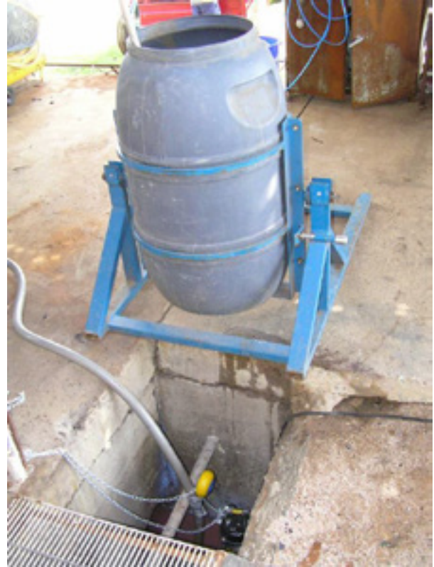
Figure 13. Tipping drum in position beside sump.
