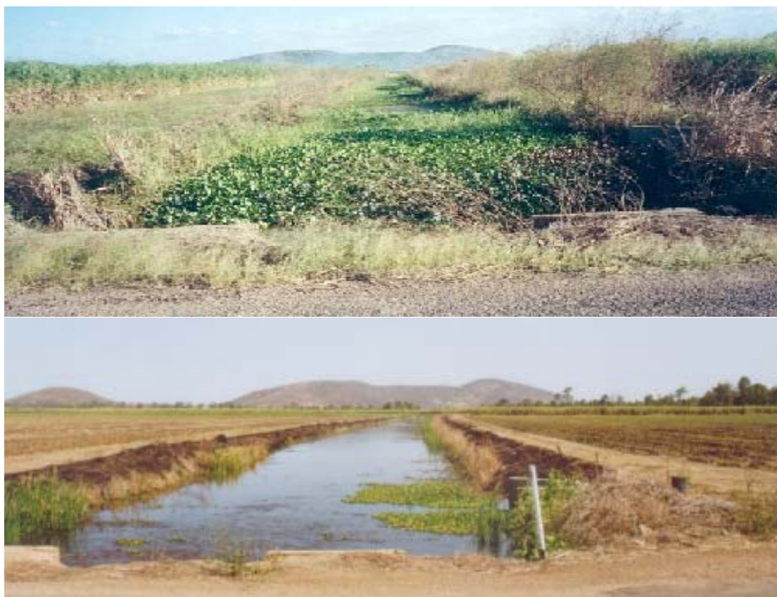
Photo 1. Sandy Creek Diversion study site: before mechanical weed harvesting (top) and after (bottom)
