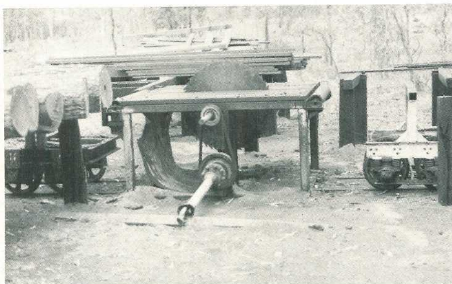
Posts are bored at the drill press as they come off the saw bench.
