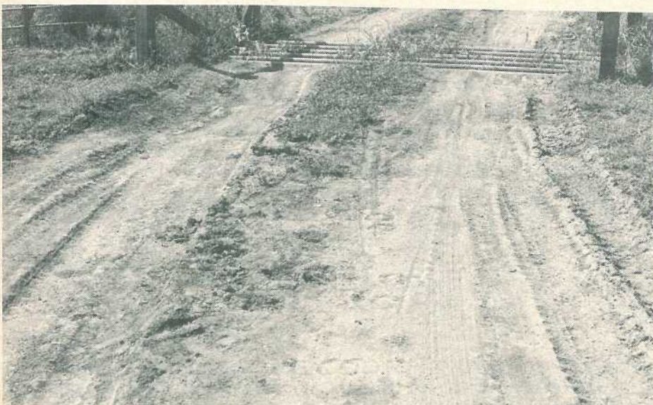
An example of pot-holing where vehicles tend to stop and start before traversing the grid.
