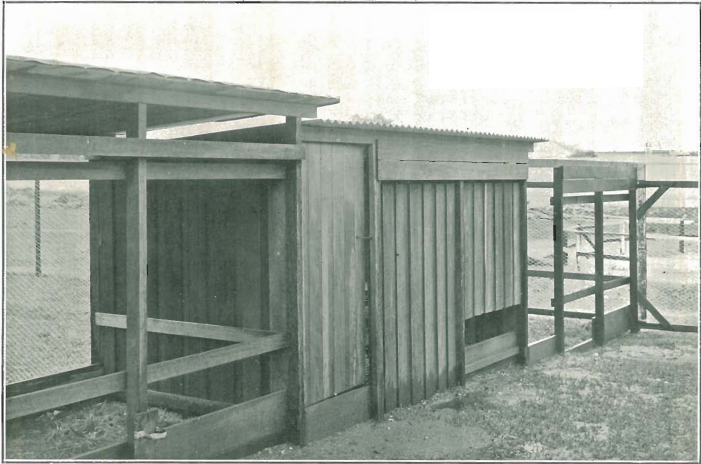
PLATE 26.—BACK VIEW, SHOWING COMPLETED HOUSE AND FRAMING WALLED WITH SAWN PALINGS.
