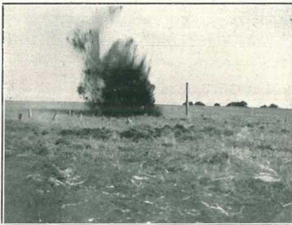
PLATE 9.—DEEP BLAST, WITH SIX PLUGS OF DYNAMITE.
