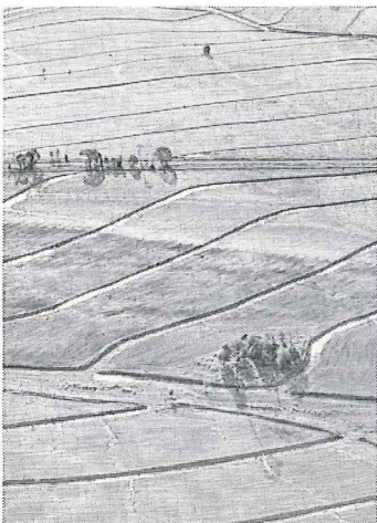
Well planned and constructed contour bank systems greatly reduced soil loss from cultivated land during the April-May 1983 rains.
