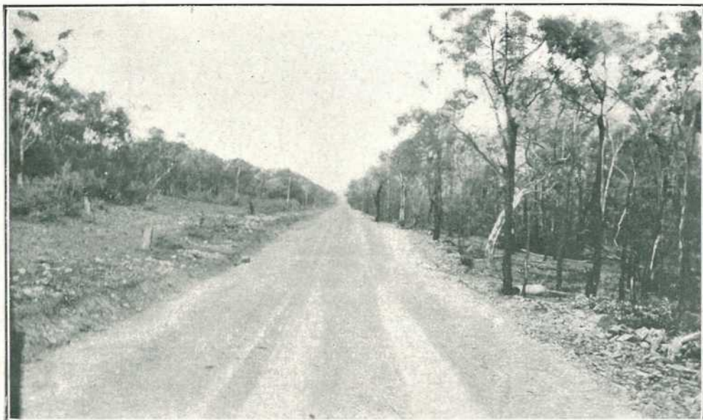
PLATE 18.—INGLEWOOD SHIRE. Gravelled section, Inglewood-Texas Road.
