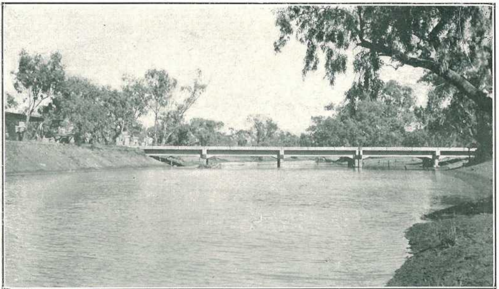
PLATE 21.—PAROO SHIRE. Low-level reinforced concrete bridge over Paroo River at Eulo, on Cunnamulla-Thargomindah Road.
