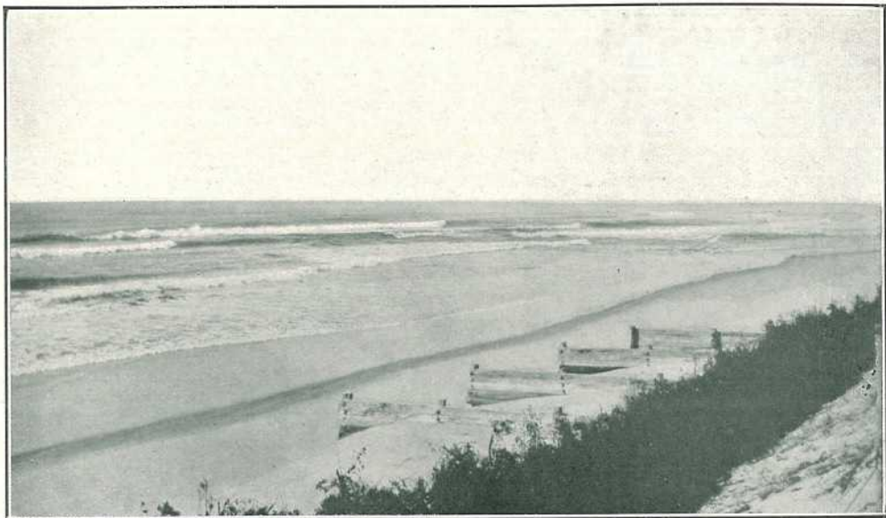
PLATE 24.—MAIN SOUTH COAST ROAD, NEAR SOUTHPORT, showing timber groynes and brush fences which have arrested wave action.
