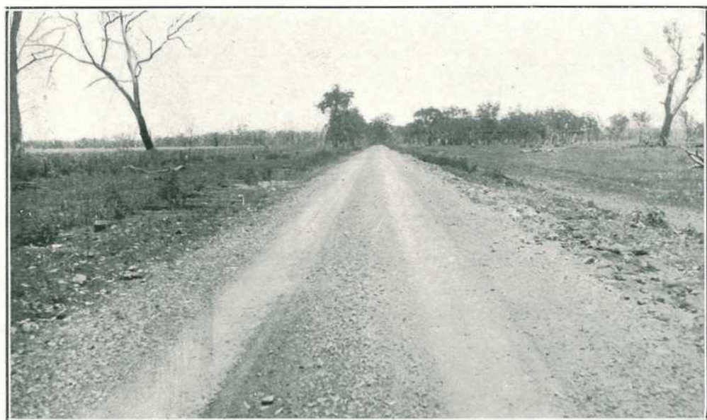
PLATE 15.—CLIFTON SHIRE. TOOWOOMBA—GOONDIWINDI ROAD. Gravelled section in the wheat area.
