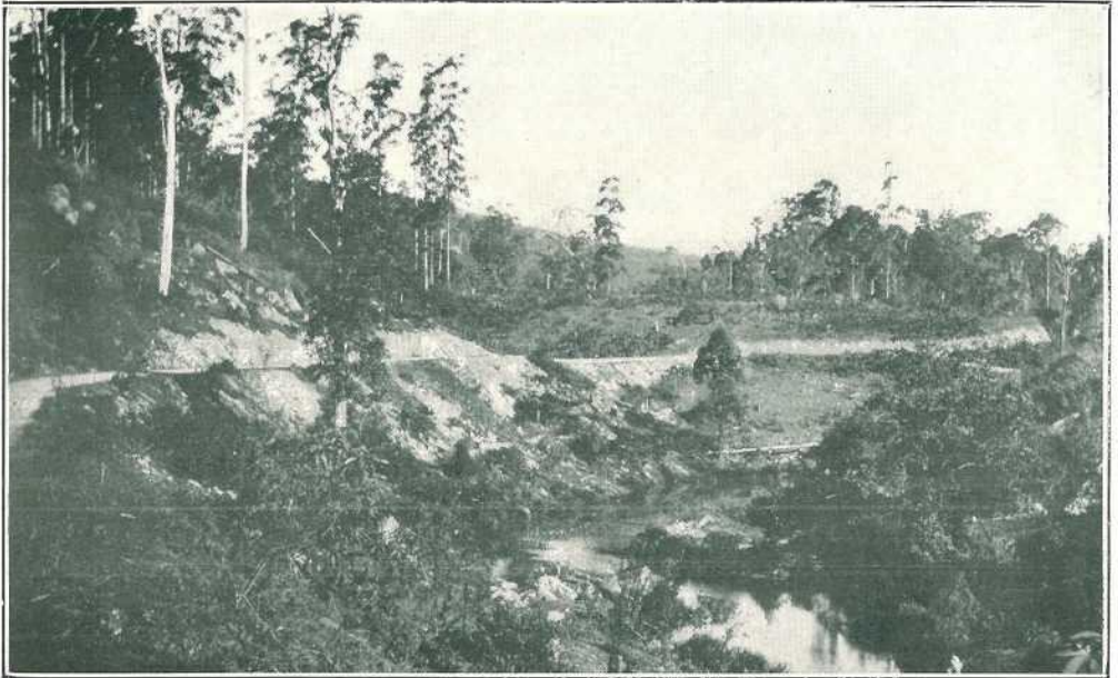
PLATE 26.—SHIRE OF NERANG. CURREMBIN CREEK DEVIATION, which eliminates several creek crossings and steep gradients.
