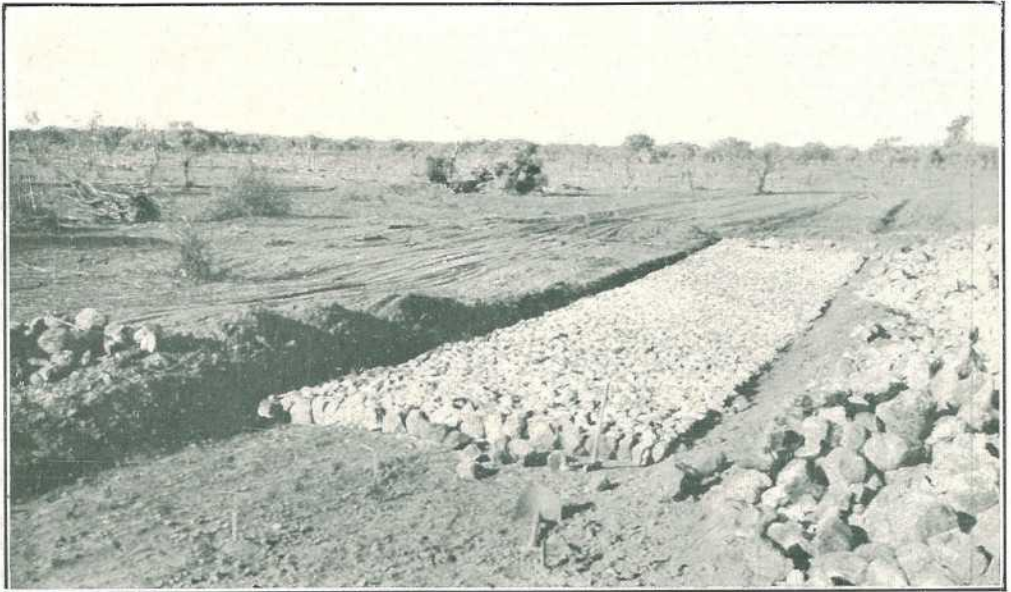
PLATE 20.—SHIRE OF BULLO. QUILPIE-EROMANGA ROAD. Typical flood invert under construction.
