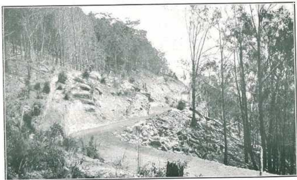
PLATE 116.—CAIRNS-TABLELAND ROAD. SECTION NEAR TOP OF RANGE.
