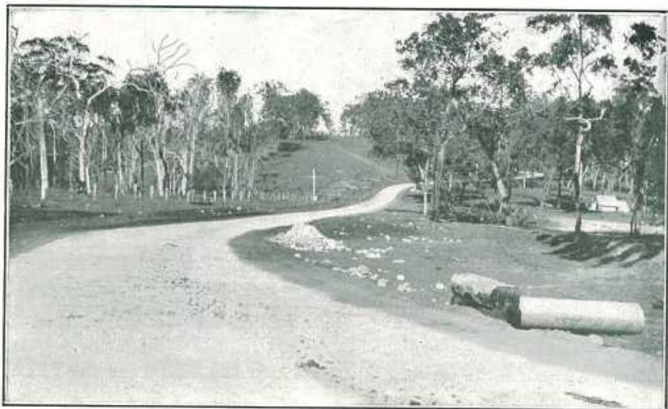
PLATE 128.—KOLAN SHIRE, GIN GIN-MIRIAM VALE ROAD, SHOWING A DEVIATION TO AVOID A STEEP GRADE.
