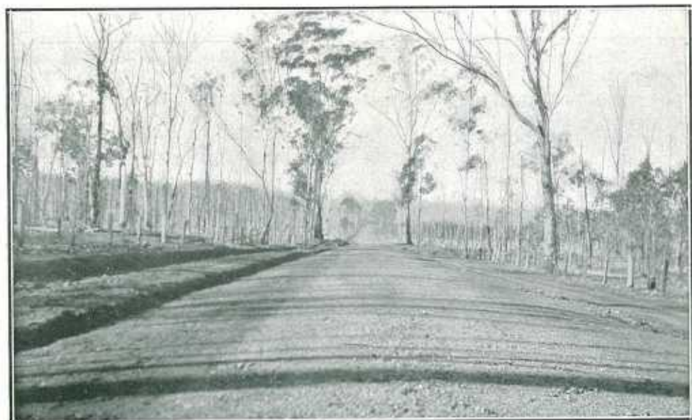
PLATE 126.—MURGOON-BARAMBAH ROAD, IN MURGOON SHIRE, LOOKING TOWARDS BARAMBAH. ROLLING INCOMPLETE.
