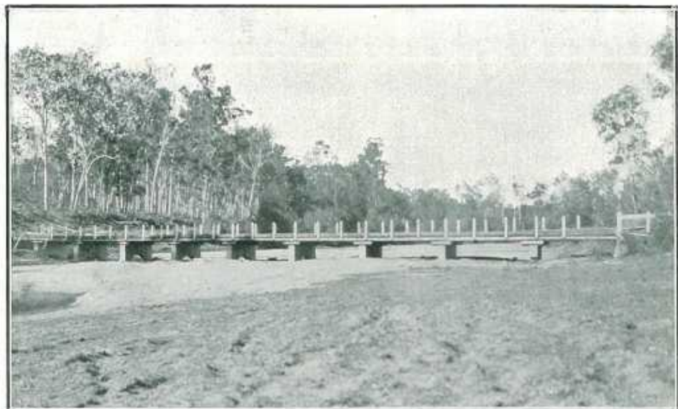
PLATE 121.—MUNDURBERRA SHIRE. LOW-LEVEL BRIDGE OVER THE BOYNE RIVER. NATIONAL GRANT PROJECT.
