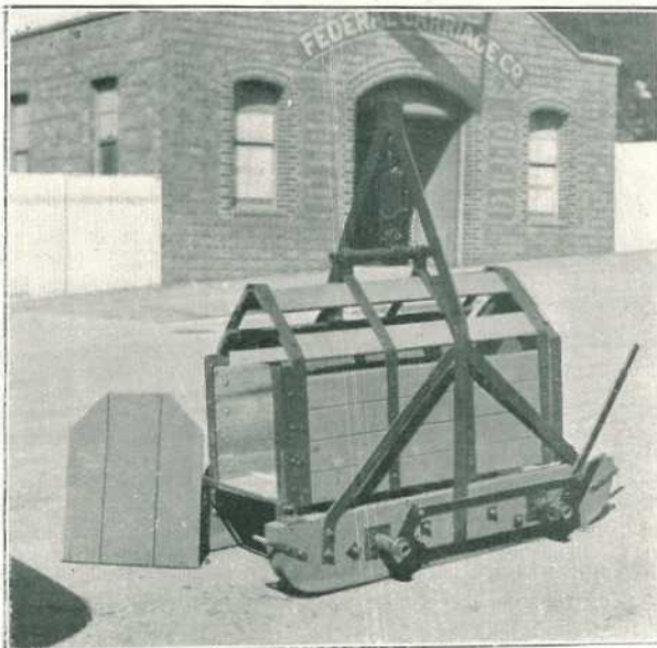
PLATE 100 (Fig. 6). Another view, showing machine ready for use and crate open ready to receive pig.
