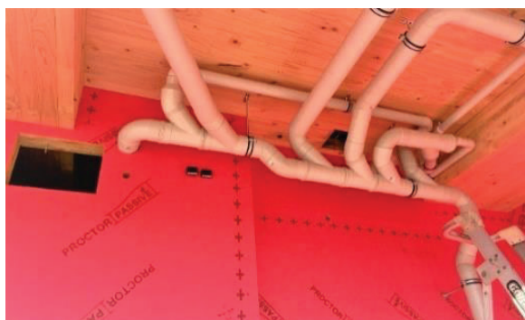
Figure 2: Sensor location close to plumbing areas on external face of the panel.
