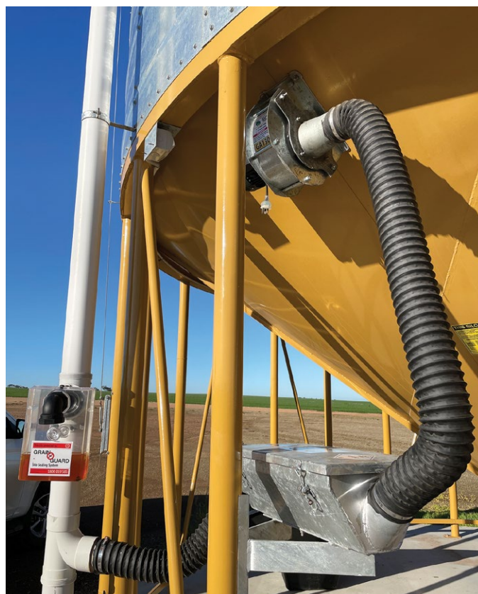
Some silos are built with a chamber and passive (thermosiphon) or powered recirculation system for applying phosphine from the bottom. Photo: Ben White, Kondinin Group
