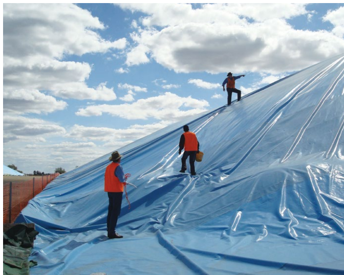
QDPI and GrainCorp staff setting up a bunker fumigation. Photo: QDPI
