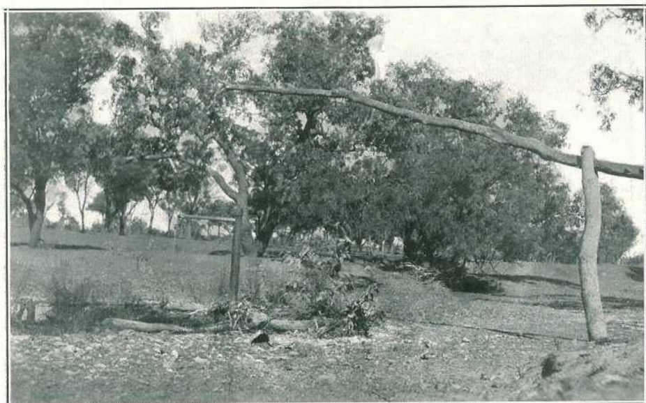
PLATE 65.—A "HAND" BORE OR BORE SUNK BY SPRING POLE METHOD IN THE NEAR WEST.
