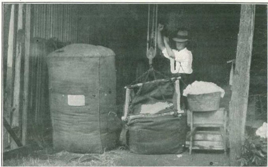
PLATE VI.—A GROWER'S APPARATUS FOR PACKING SEED COTTON IN A WOOL-PACK.
