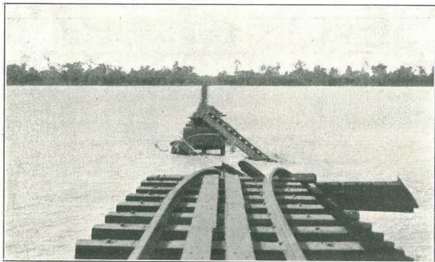
PLATE 19.—DAMAGE DONE TO RAILWAY BRIDGE OVER THE BURDEKIN RIVER BY FLOOD, 1916 (SOUTHERN END).
