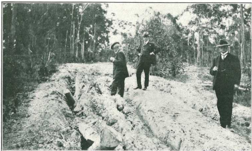
PLATE 34.—SHOWING DAMAGE TO ROAD BY BAD FOUNDATION AND EXCESSIVE LOADS.
