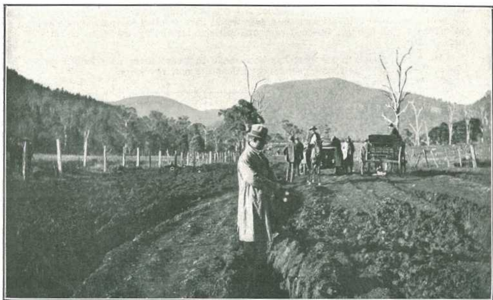
PLATE 31.—BLACKSOIL ROAD ON THE DARLING DOWNS CUT UP BY WHEEL TRAFFIC DURING WET WEATHER.
