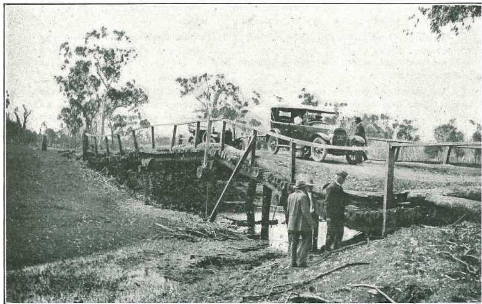
PLATE 38.—BRIDGE IN A BAD STATE THROUGH NEGLECT OF MAINTENANCE.
