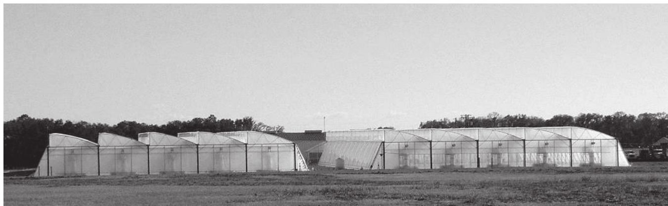
Fig. 3. Passively ventilated greenhouses at the Protected Agriculture Center in Gainesville, Fla. The greenhouse units used in the budget analysis presented in this report were similar but with a larger area.
