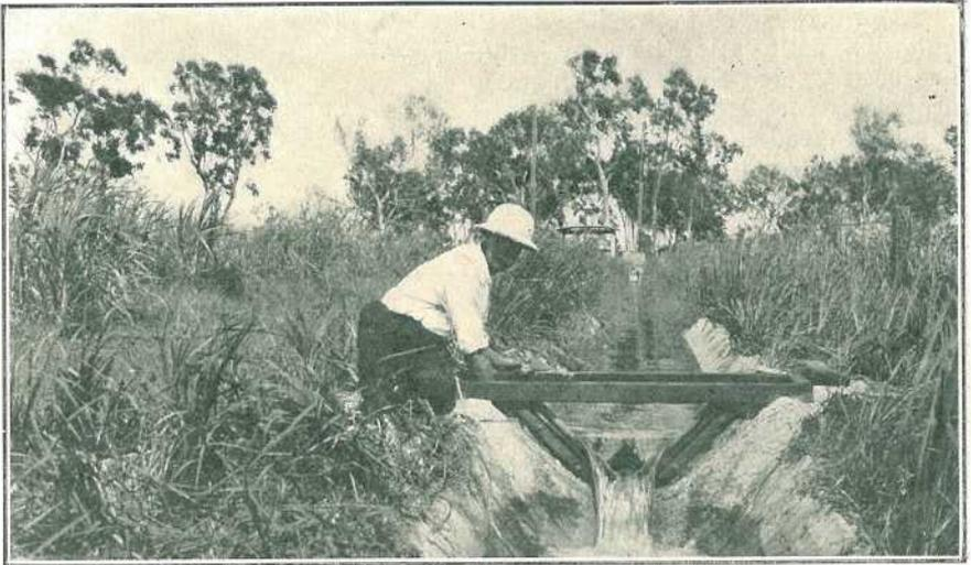
PLATE 6.—CONCRETE-LINED CHANNEL, LEADING FROM NO. 1 WELL, LENNOX'S BLOCK.
