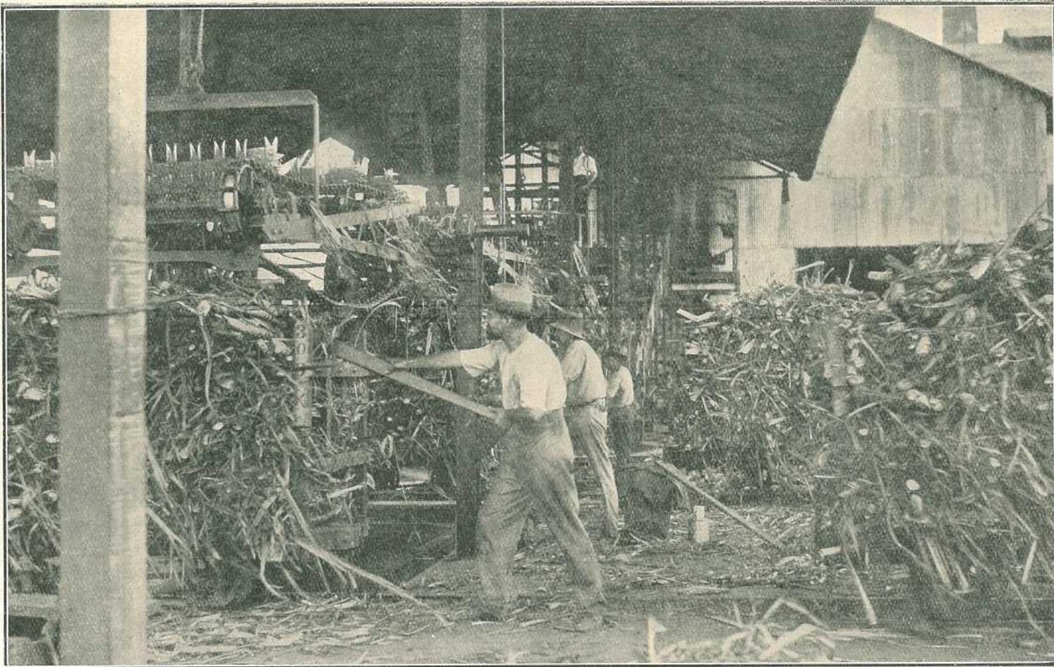
PLATE I.—FEEDING CANE TO THE CARRIER, SOUTH JOHNSTONE SUGAR MILL.
