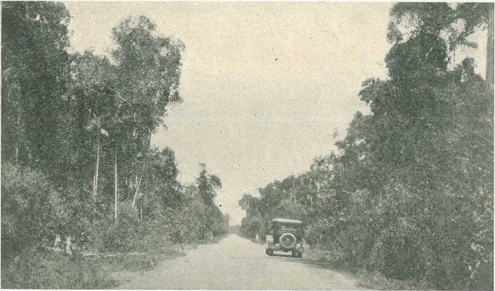
PLATE 153.—CARDWELL SHIRE—TULLY RIVER-NORTH BANK ROAD. The luxuriant tropical foliage abutting the road has been preserved in its virgin state. The road serves a sugar district and a seaside resort.
