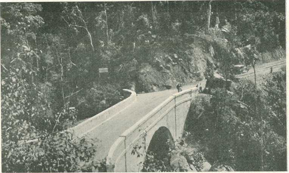
PLATE 154.—THURINGOWA SHIRE—MOUNT SPEC ROAD. A masonry arch bridge built entirely by relief workers.
