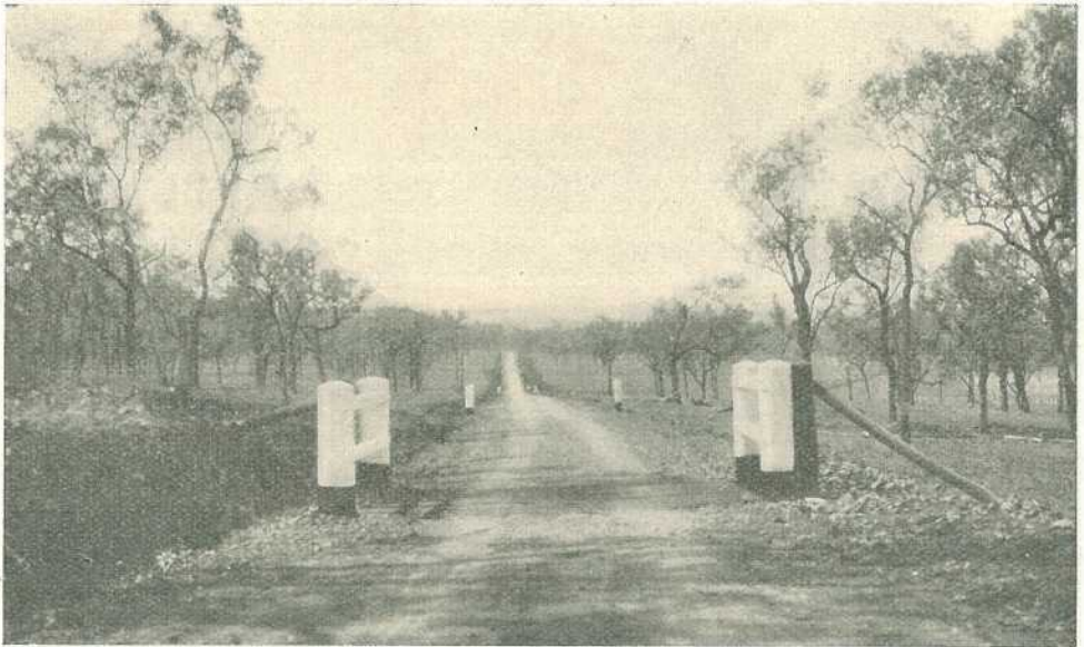
PLATE 163.—MONTOSHIRE—MONTOSH-THANGOO ROAD. A standard type of M.R.C. cattle grid near Coomingleh.
