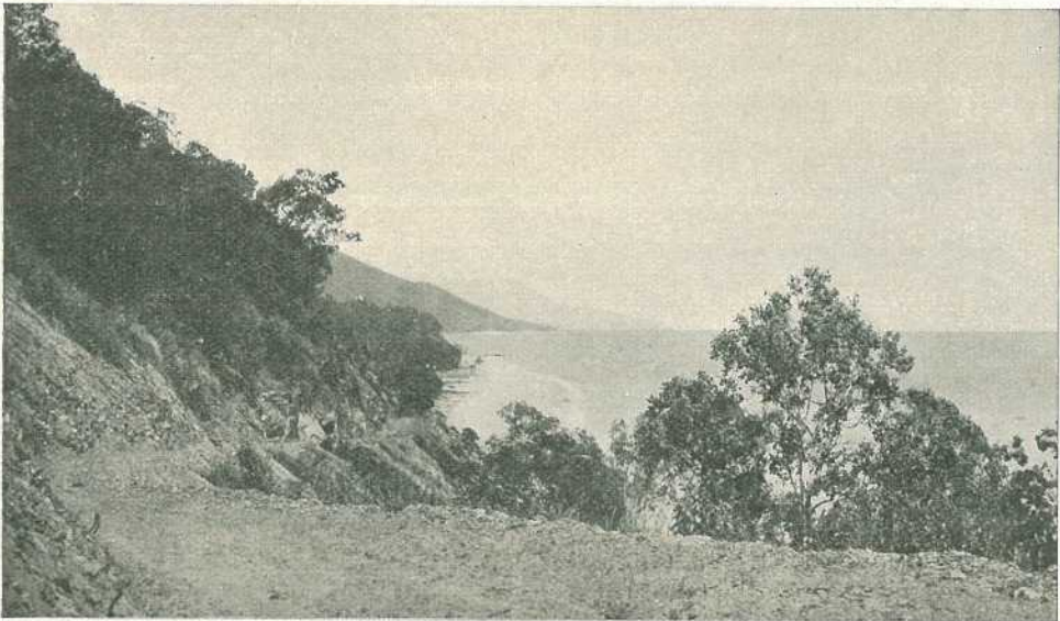
PLATE 149.—CAIRNS-PORT DOUGLAS ROAD UNDER CONSTRUCTION.
