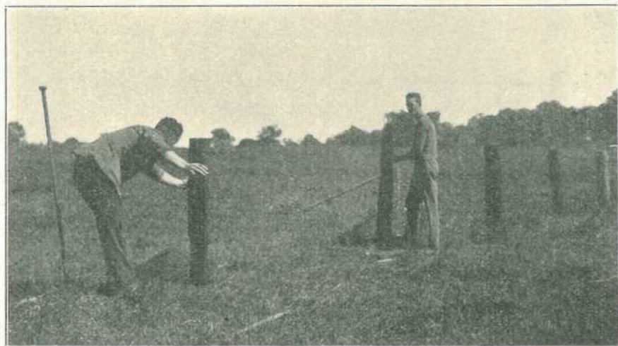
PLATE 38.—SIGHTING A LINE OF FENCING. Example of practical instruction at St. Lucia Farm School.
