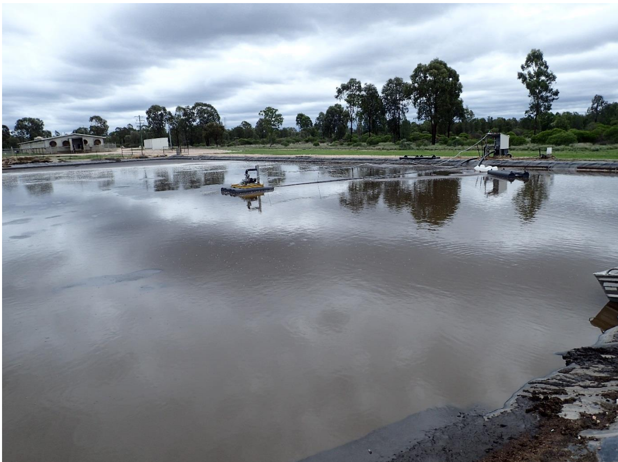
Figure 38 Pond 2 (Piggery A) showing the pontoon mounted pump used to transfer effluent to a secondary pond.
