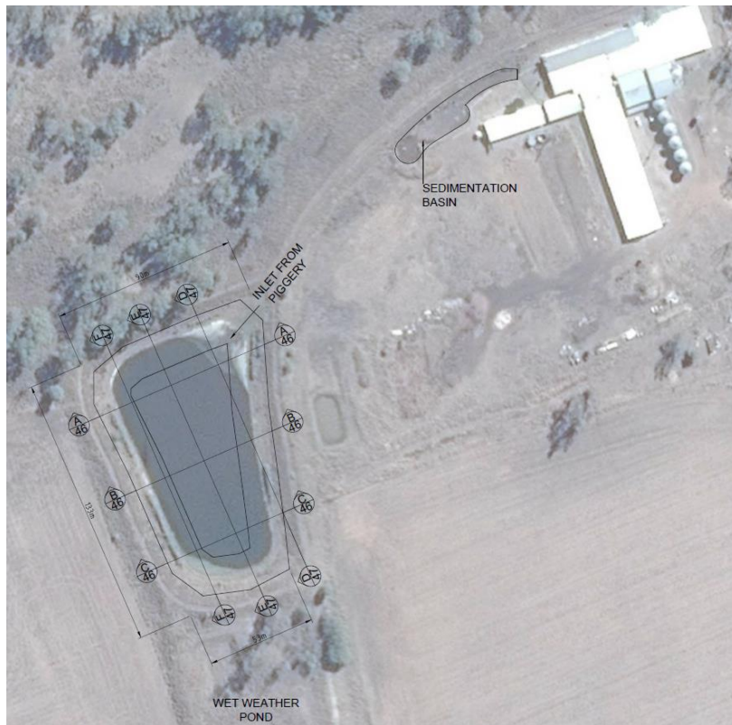
Figure 29 Aerial photograph of Piggery G, Pond 12.
