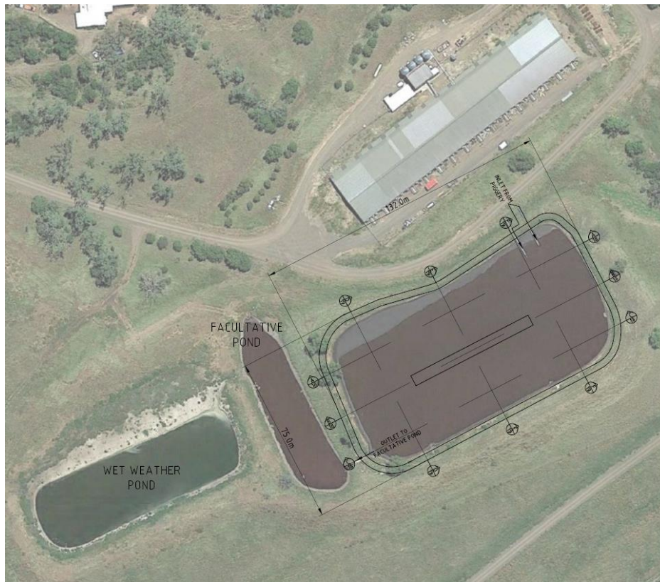
Figure 17 Aerial photograph of Piggery C, Pond 6.
