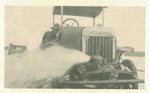
PLATE 14.—JETTING CONCRETE PILES.
