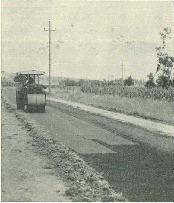
PLATE 63. BRISBANE-TOOWOOMBA ROAD. Rolling and smoothing after drag operations.
