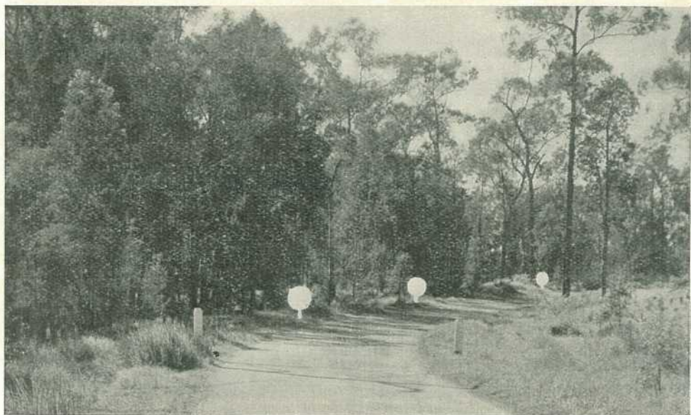
PLATE 59. PACIFIC HIGHWAY (MAIN SOUTH COAST ROAD). Night visibility discs on curves.
