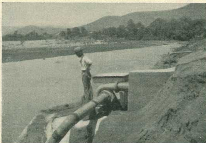
PLATE 47.—SHOWING CENTRIFUGAL PUMP.
