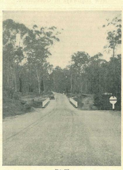
Plate 352. LANDSBOROUGH SHIRE.—Bruce Highway Tourist Road (Landsborough-Beerwah Section). Two 3/30-feet span timber bridges over Back Creek.
