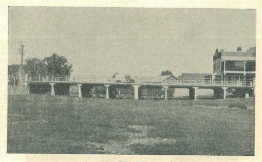
Plate 357. Bridge over Bradley's Gully on the Charleville-Adavale Road at Charleville. This modern reinforced concrete slab bridge replaced an old timber structure.
