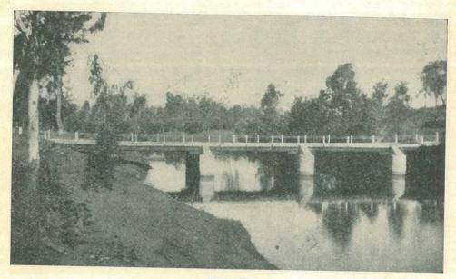
Plate 366. BANANA SHIRE.—Dululu-Bunerba Road. Bridge over Dee River, timber superstructure, bitumen deck-wearing surface on concrete cylinders.
